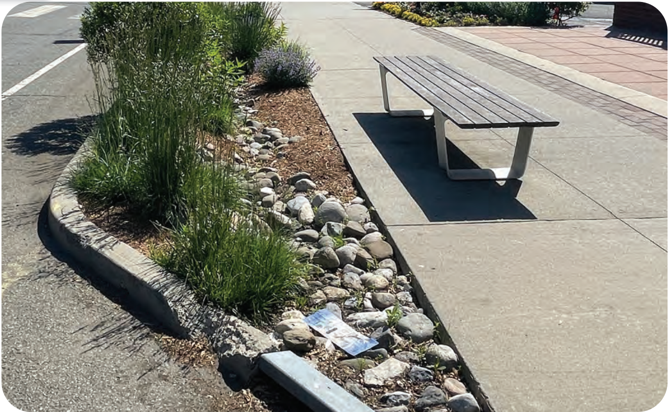
Complete Street with rain garden in curb extension, and sidewalk seating in Millburn, NJ
