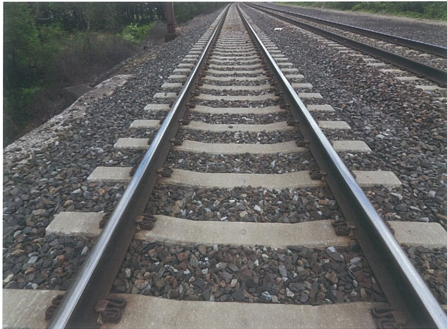
PHOTO 5-5: General view of bridge ties, Track #2, looking west.
