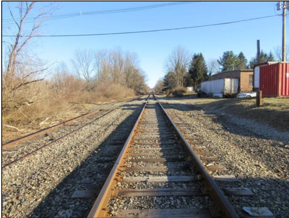
Figure 4.4: West Approach – Looking East
