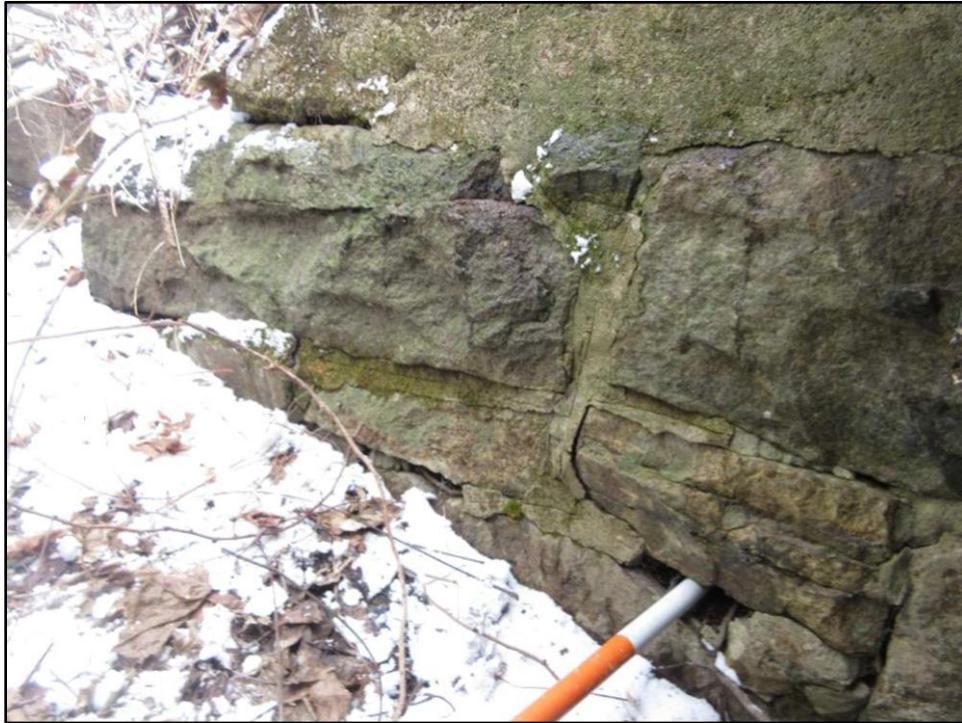
Figure 4.9: Northeast Wingwall – Looking Northeast
