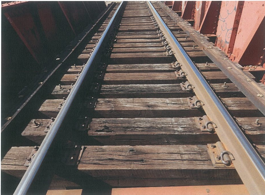
PHOTO 5-5: General view of bridge ties, Track #1, looking west.
