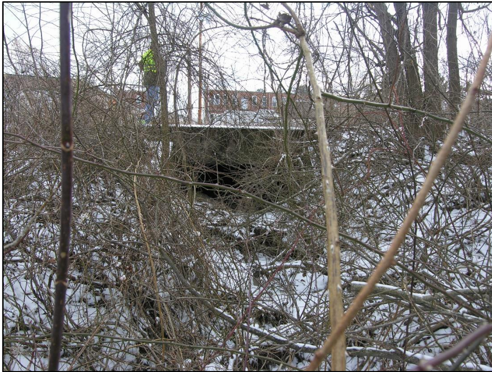
Figure 4.10: Headwall – Northwest End – Looking Southwest
