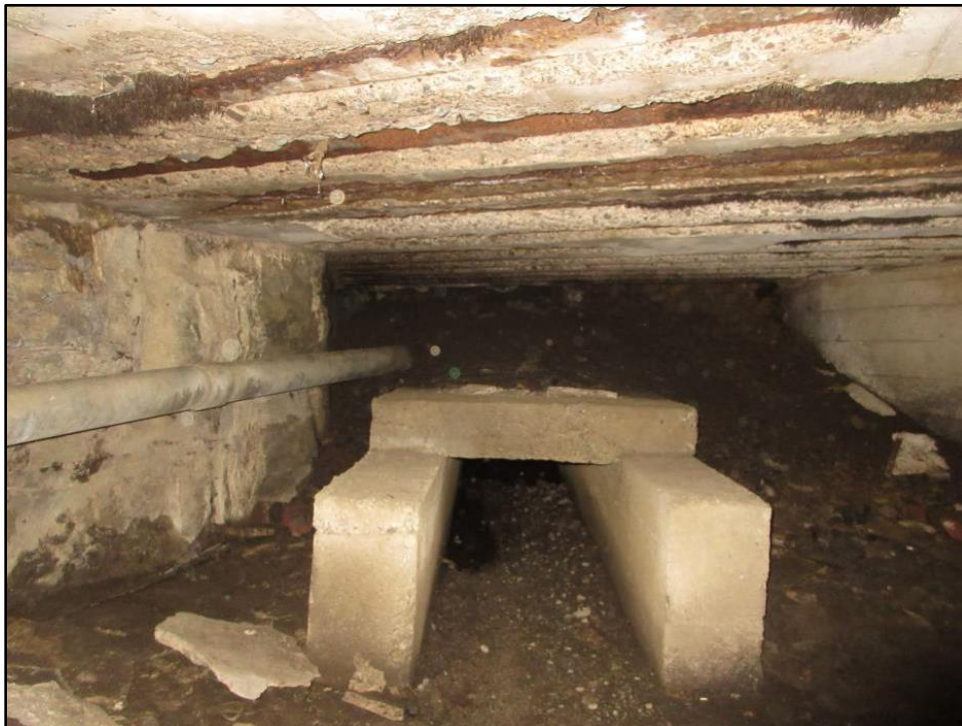
Figure 4.11: Southeast End of Culvert – Looking Southeast
