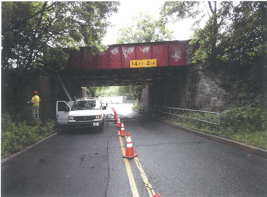
PHOTO 5-1: South elevation, looking north. Work Done: 14'-2" Vertical clearance sign has been installed at the south fascia.
