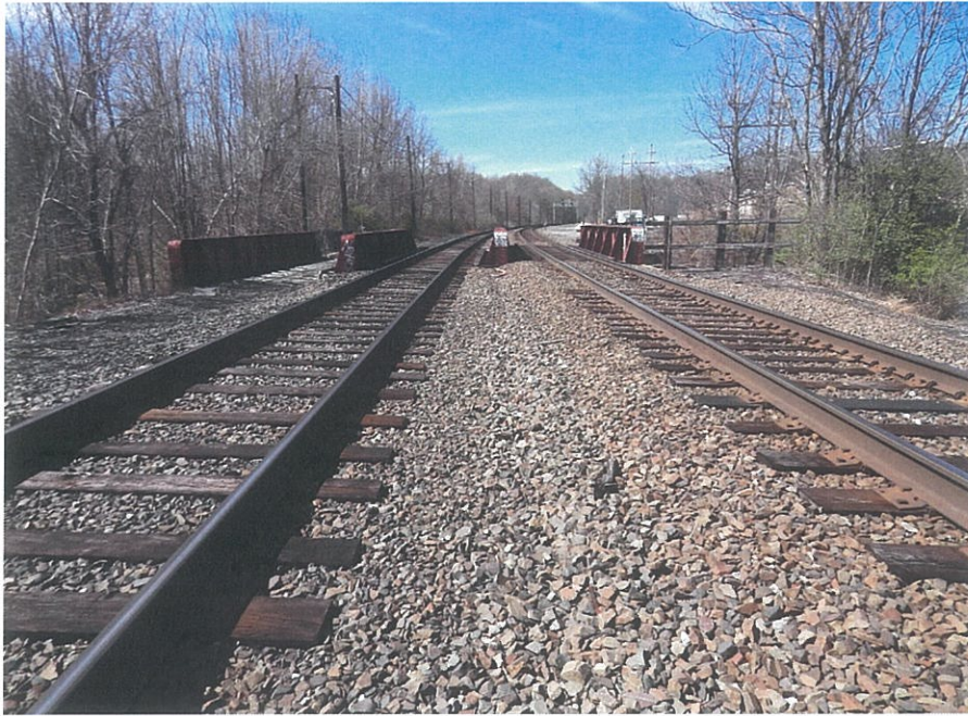
PHOTO 5-3: East approach, looking west.
