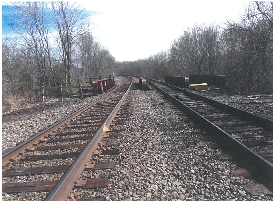
PHOTO 5-4: West approach, looking east.
