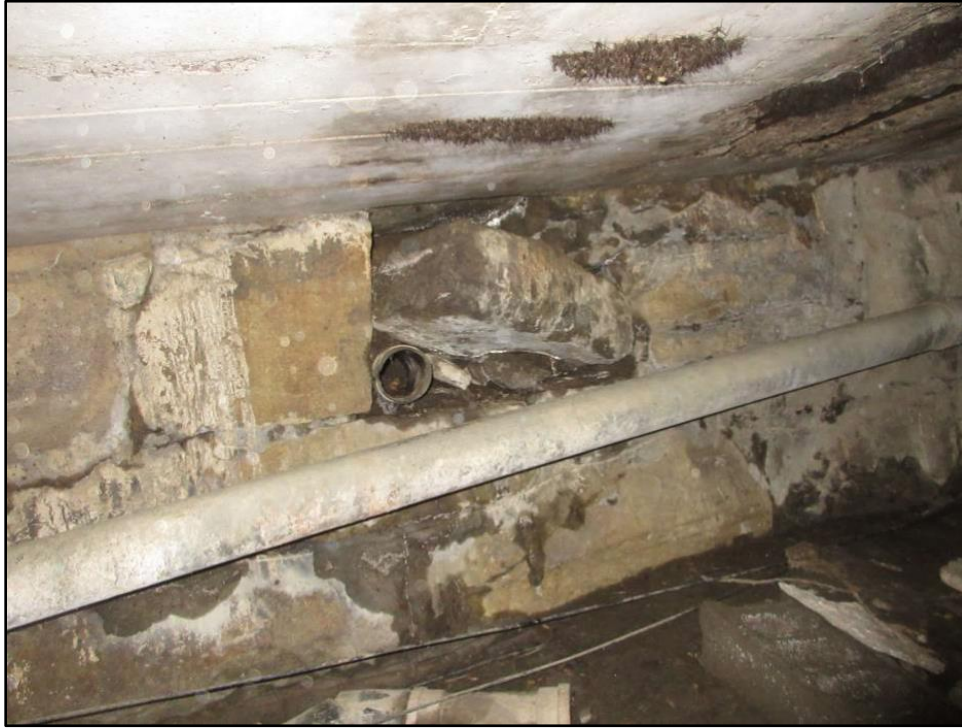
Figure 4.8: East Abutment – Looking Southeast
