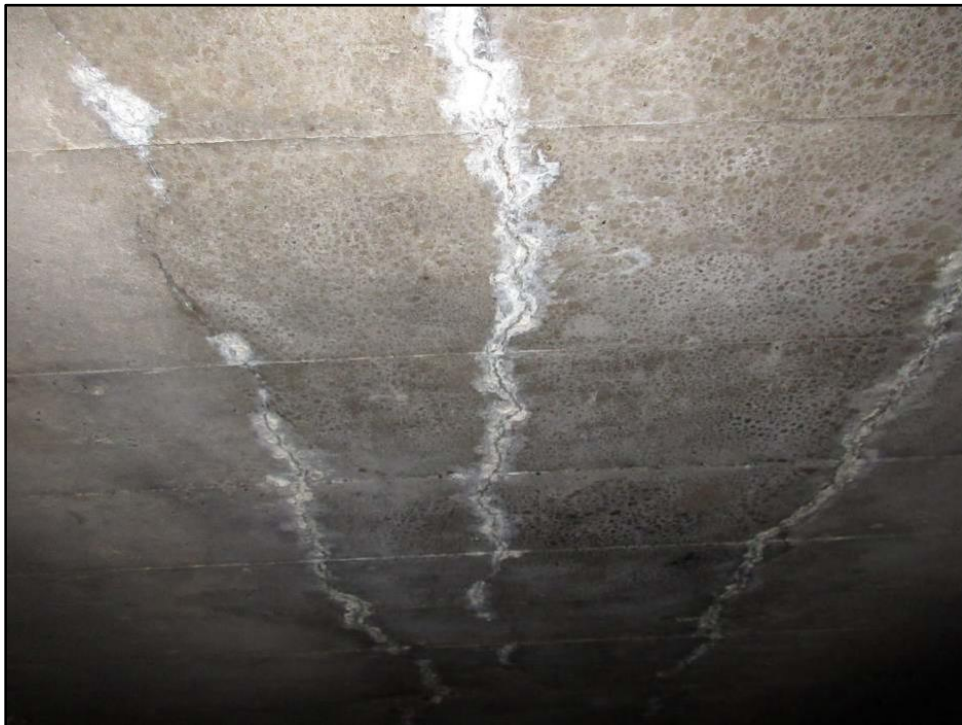
Figure 4.7: Underside of Concrete Slab – Looking Southeast
