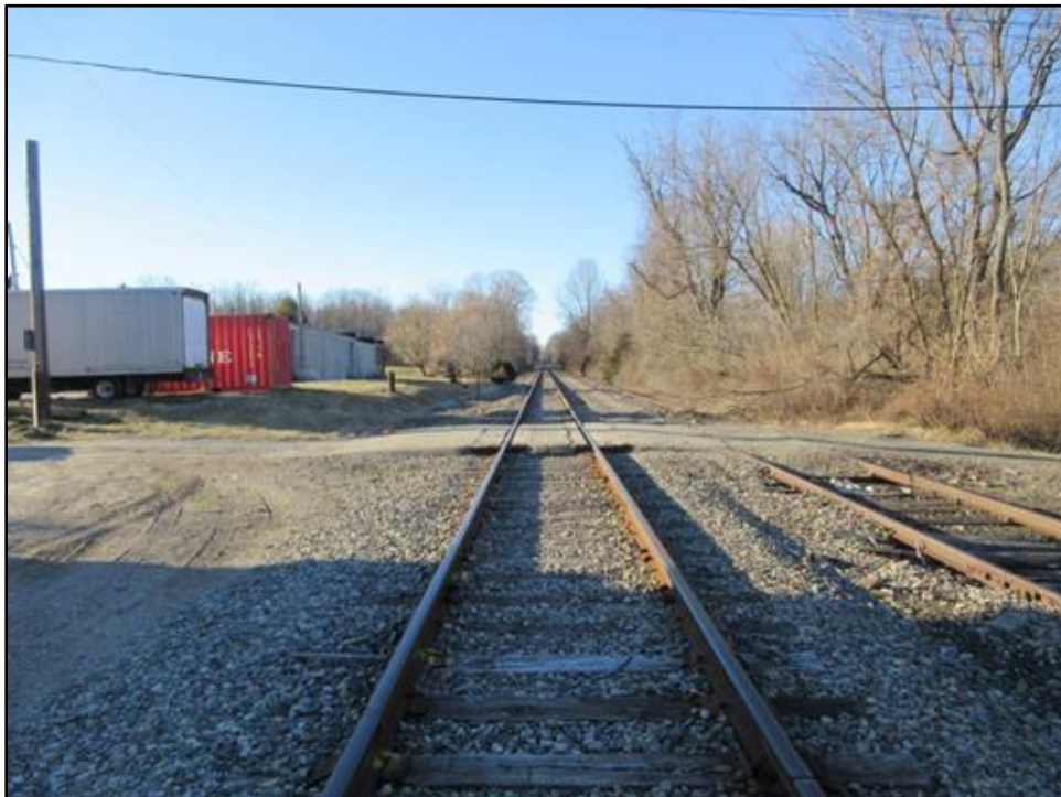
Figure 4.5: East Approach – Looking West
