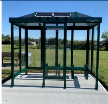
Figure 15: NJ TRANSIT's new solar-powered shelters have lighting and charging ports for electronic devices. (Image Source: NJ TRANSIT)
