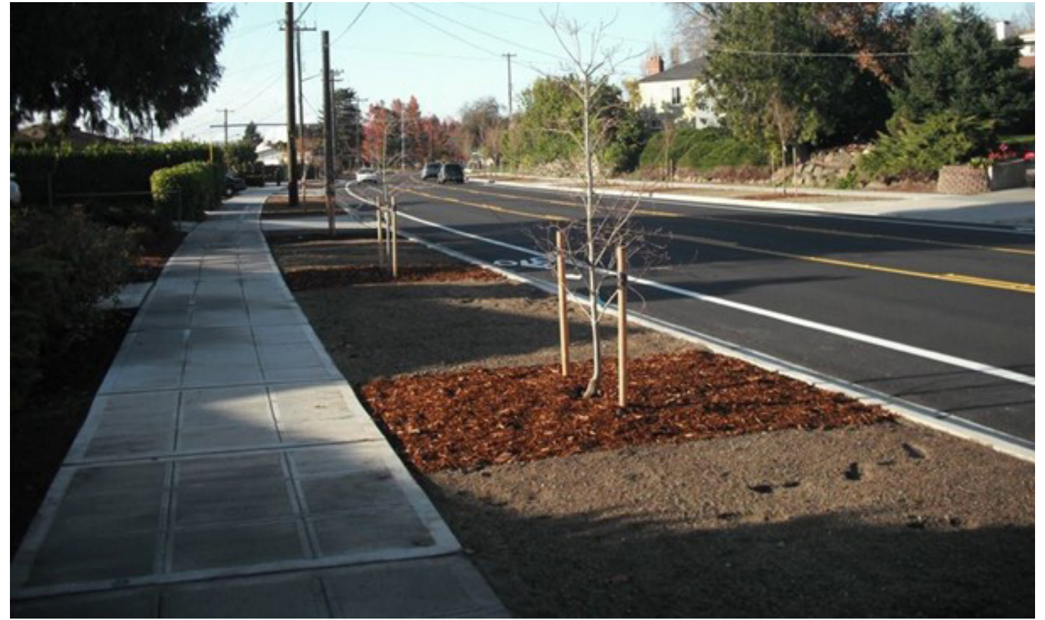
Figure 5: Wide sidewalks with a generous buffer provides a more pleasant walking experience. Buffer areas like the one shown in this photo can be used for other community-enhancing amenities such as street trees, landscaping, and green storm water management. (Image Source: NACTO)
