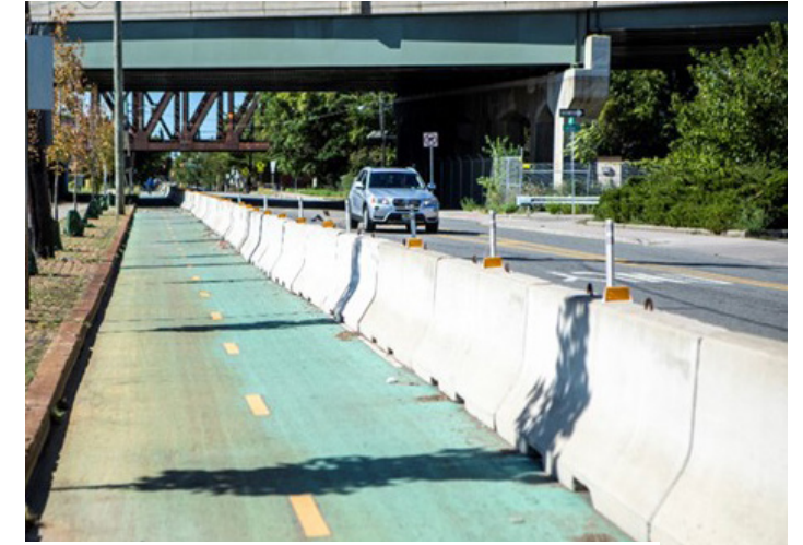
Cycle Track protected by Jersey Barrier
