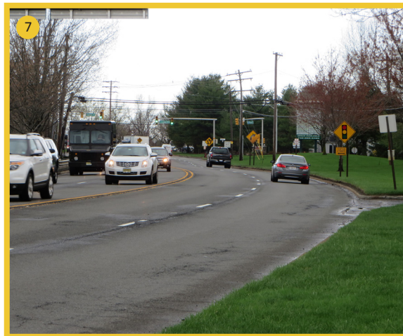
There is no edge-of-pavement line
