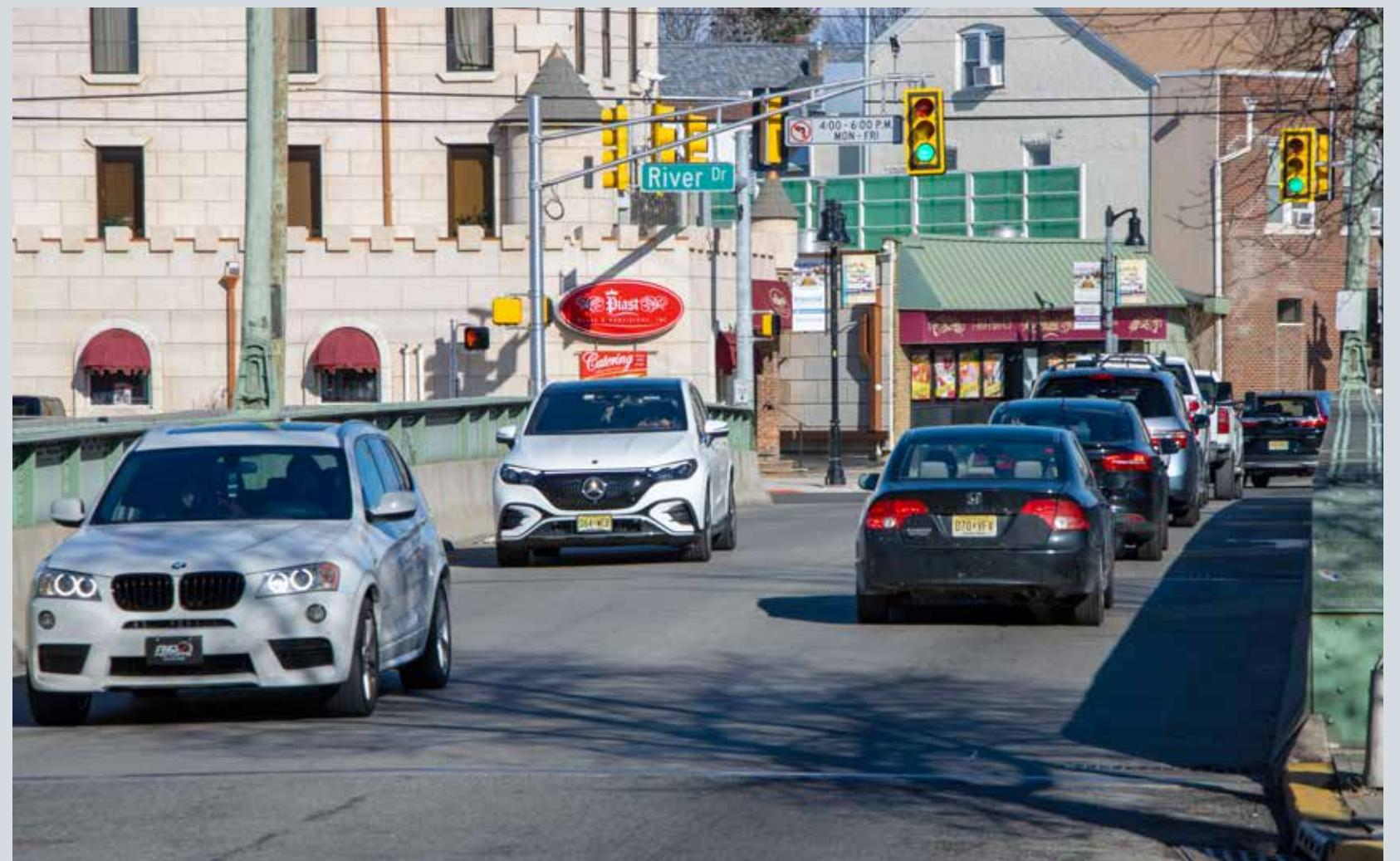
travel lane in each direction and sidewalks on both sides. On average, more than 11,000 vehicles use the bridge each day. The Passaic Street Bridge experiences significant traffic and its width is inadequate to meet current and projected vehicle and bicycle volumes. In addition, the bridge deck is below the flood elevation, according to the Federal Emergency Management Agency.
