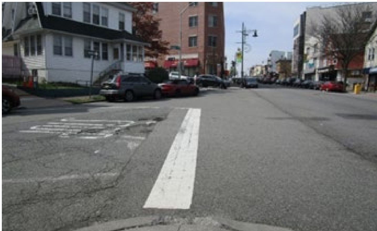
FIGURE 32. CURRENT CONDITION AT THE SOUTHERN CORNER OF MAIN & EAGLE.
