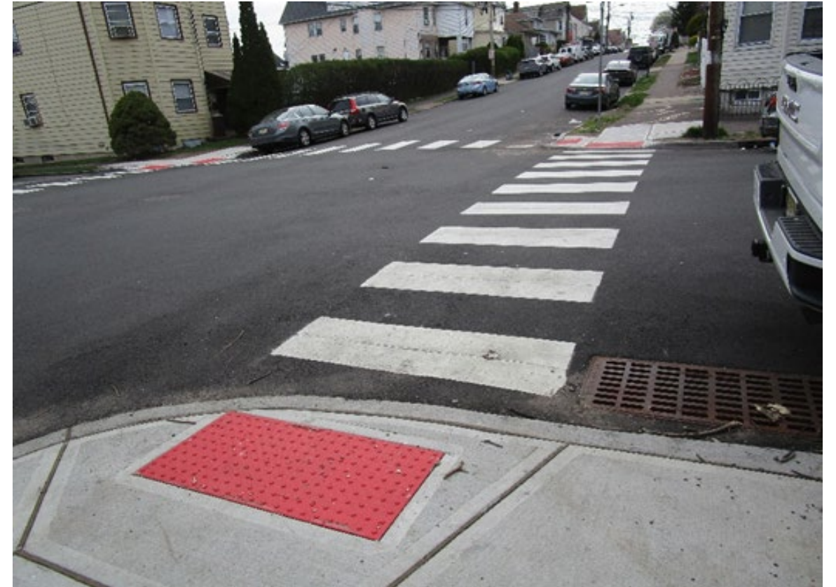
FIGURE 5. SEVERAL CROSSWALKS AROUND MAIN & EAGLE TRIANGLE PARK HAVE BEEN RECENTLY UPDATED AND ARE BOTH HIGHLY VISIBLE AND ADA ACCESSIBLE.
