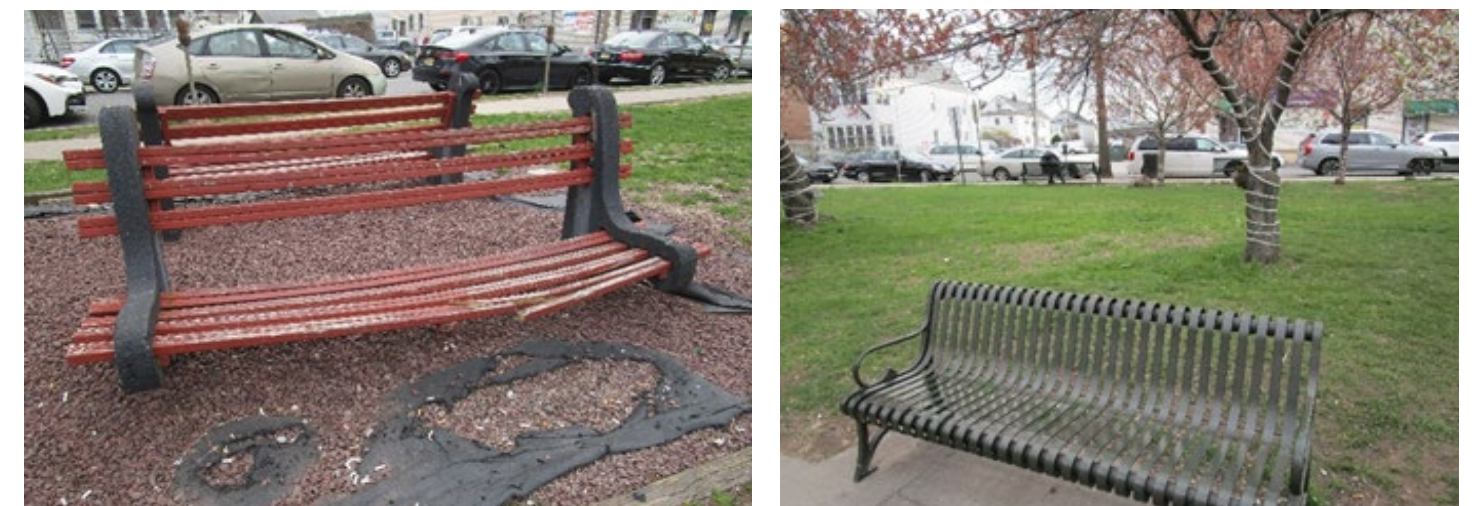
FIGURE 18. (LEFT) THE BROKEN BENCH, UNEVEN PAVEMENT AND WOODEN PERIMETER MAKES USING THESE BENCHES CHALLENGING AND UNSAFE. (RIGHT) THE BENCHES ALONG THE PARK'S PERIMETER ARE IN GREAT CONDITION.
