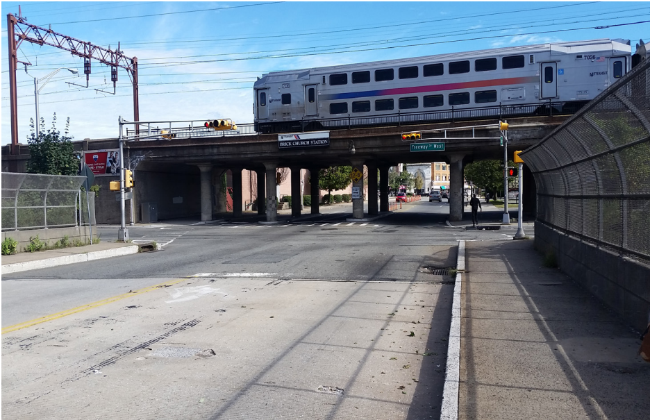
Brick Church Station – South Harrison Street underpass
