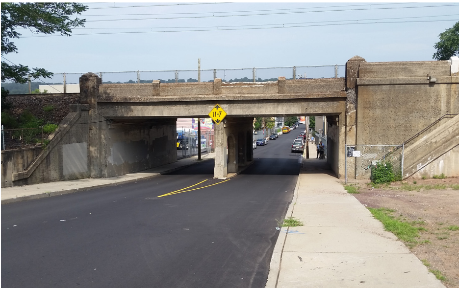
Highland Avenue Station – Freeman Street underpass
