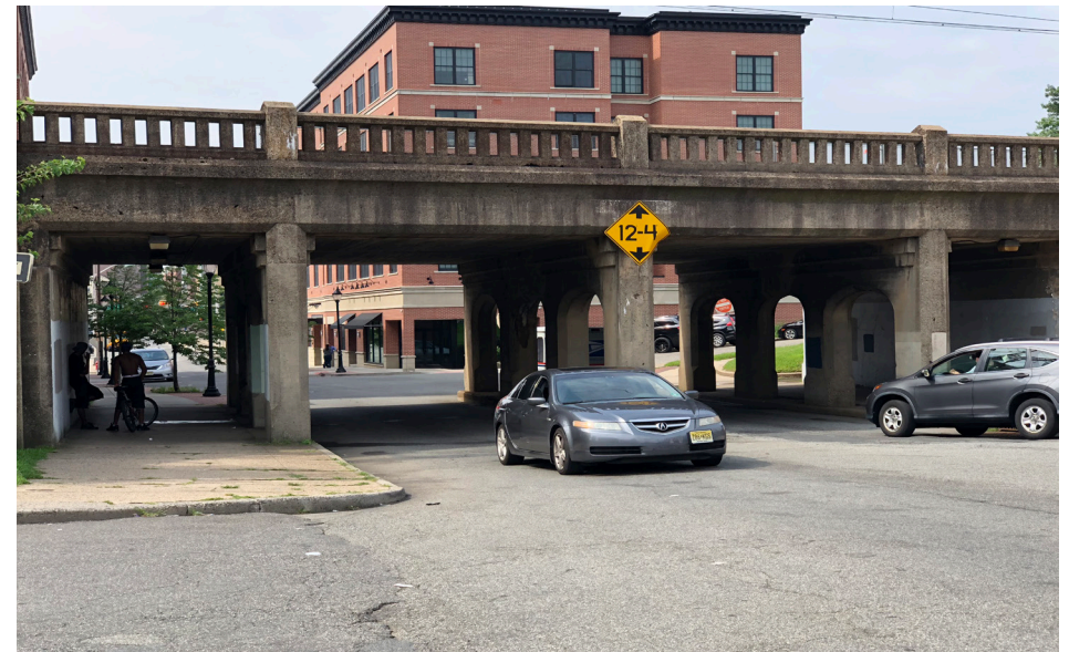
Orange Station – South Essex Avenue underpass
