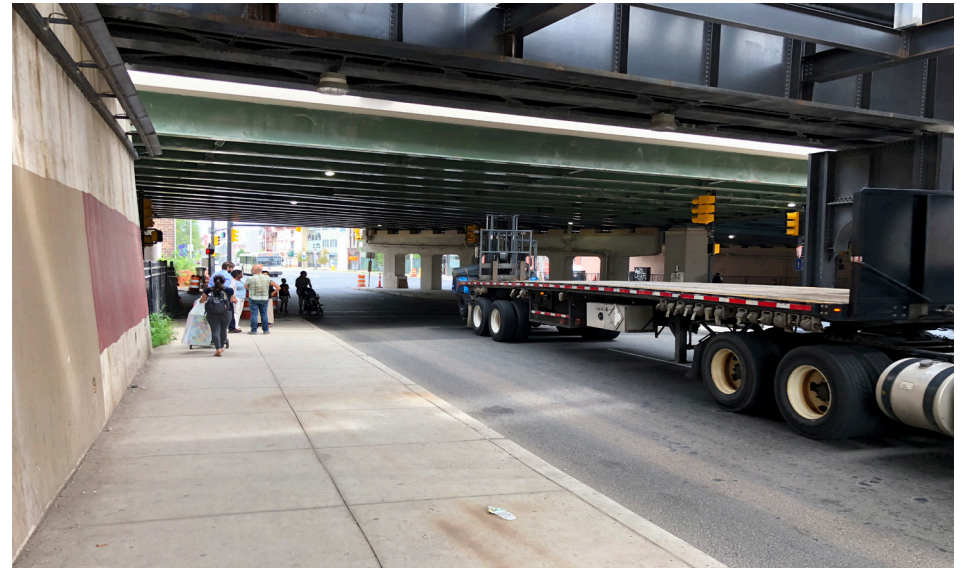
Newark Broad Street Station – Broad Street underpass ( includes I-280)
