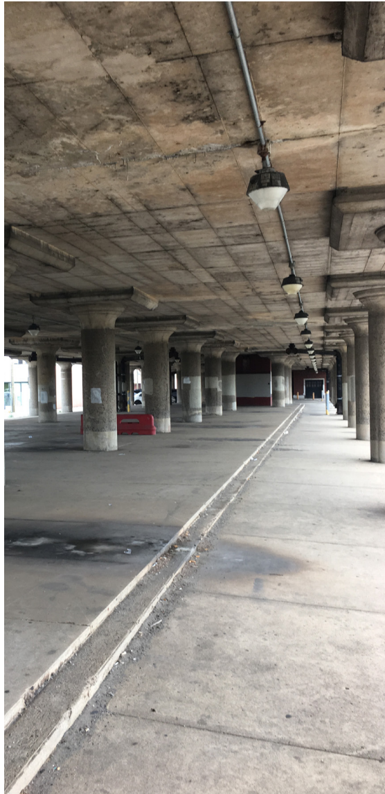
Brick Church Station underpass
