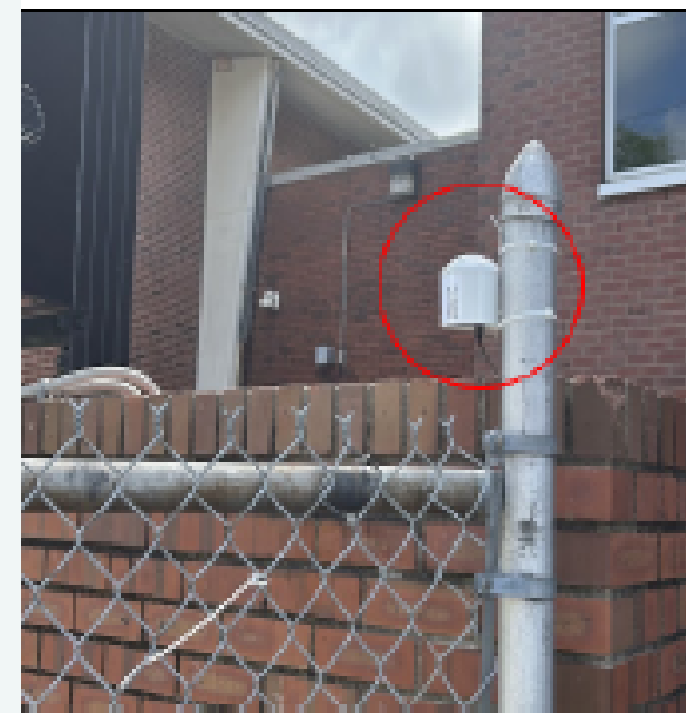
Figure 3. Air Quality Monitor Placement Close Up - Front of School.
