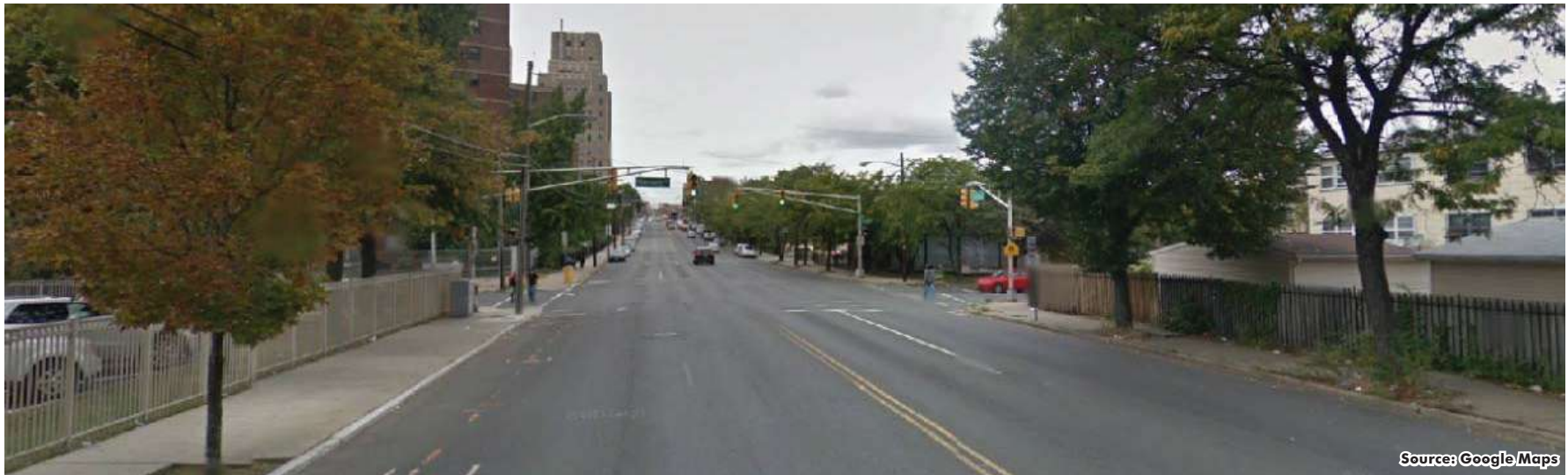
Montgomery Street at Florence Street - looking West
