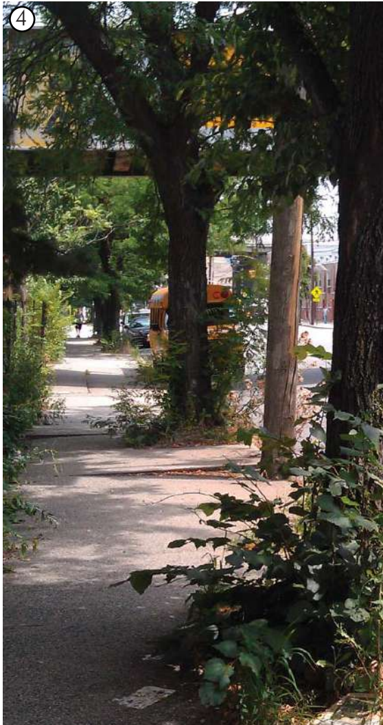
Many sidewalks need widening, repair, & better, regular maintenance
