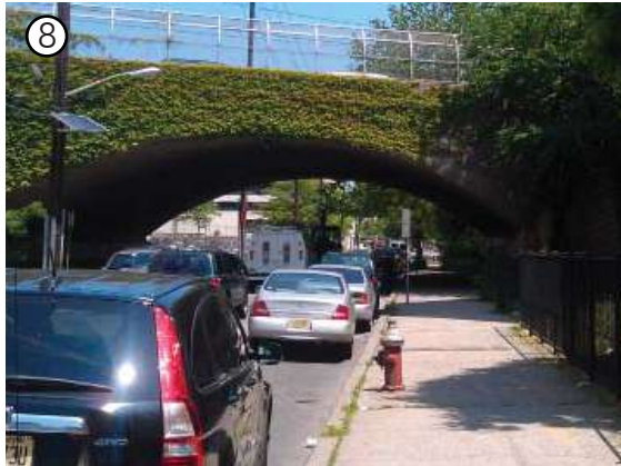
8 Cornelison underpass is dark & perceived unsafe, creating difficult cross connections
