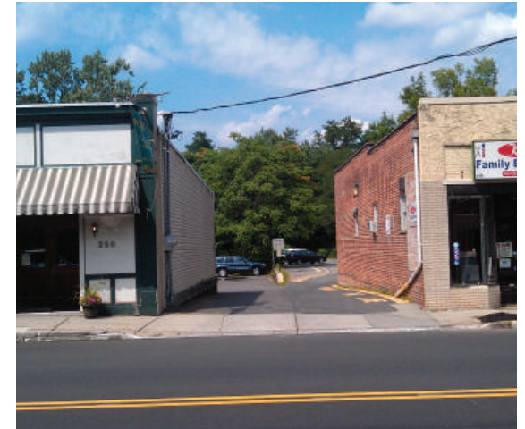
Parking is generally located behind buildings with many curb cuts along Morris Avenue
