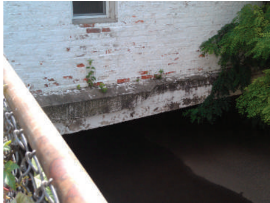
Van Winkle traveling under building
