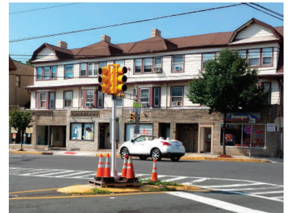
Temporary traffic signals on Morris and Mountain Avenues
