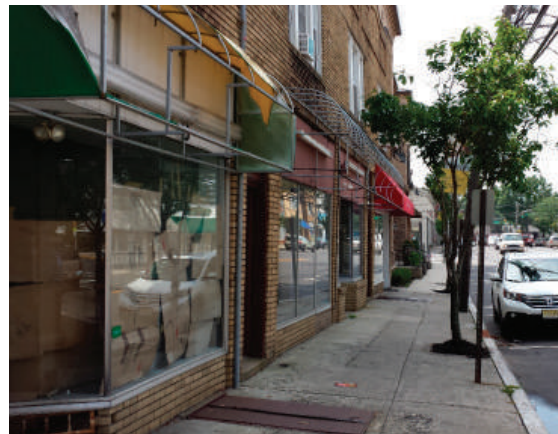
Poorly maintained awnings and sidewalks
