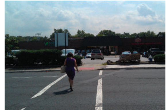
Many crosswalks and traffic stripes are in need of repainting and lack adequate signage
