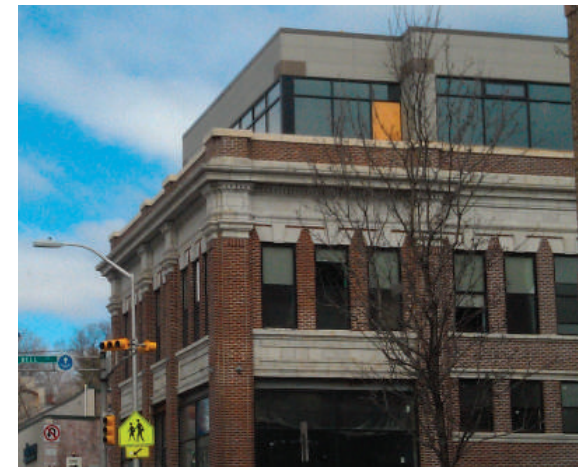
An expression line with a cornice and parapet allows a loft while maintaining the scale of the street
