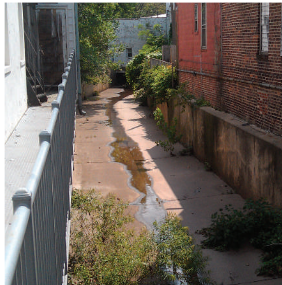
Van Winkle Brook is channelized through much of the Study Area and is prone to flooding
