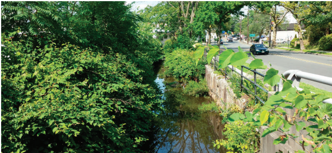
Open portion of Van Winkle Brook along Mountain Avenue
