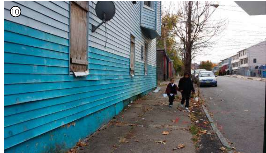
Abandoned and boarded-up buildings create a harsh & unsafe streetscape lacking visibility both to and from the street
