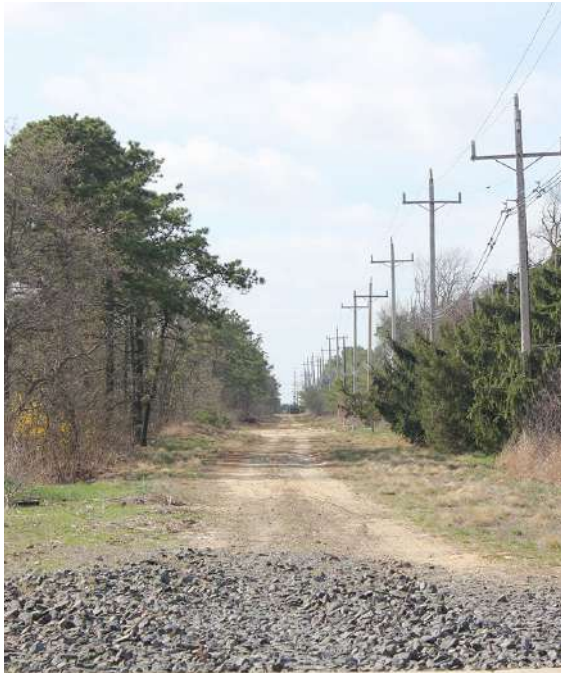
Existing Rail ROW Parallel to Route 37
