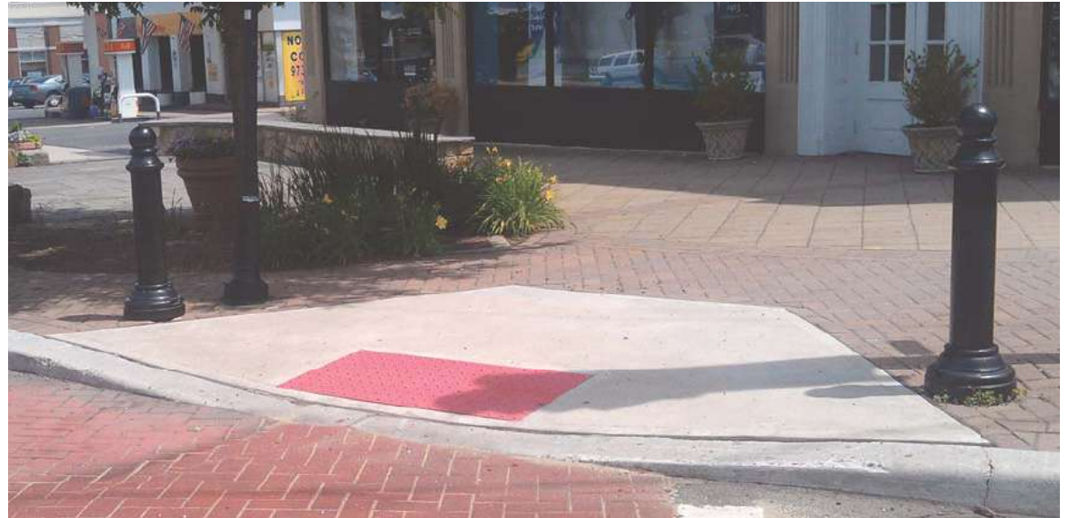
Protective bollards at the corner
