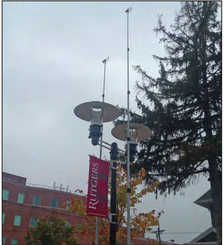
Figure 11. Video Camera Rig (Attached to Street Lighting)
