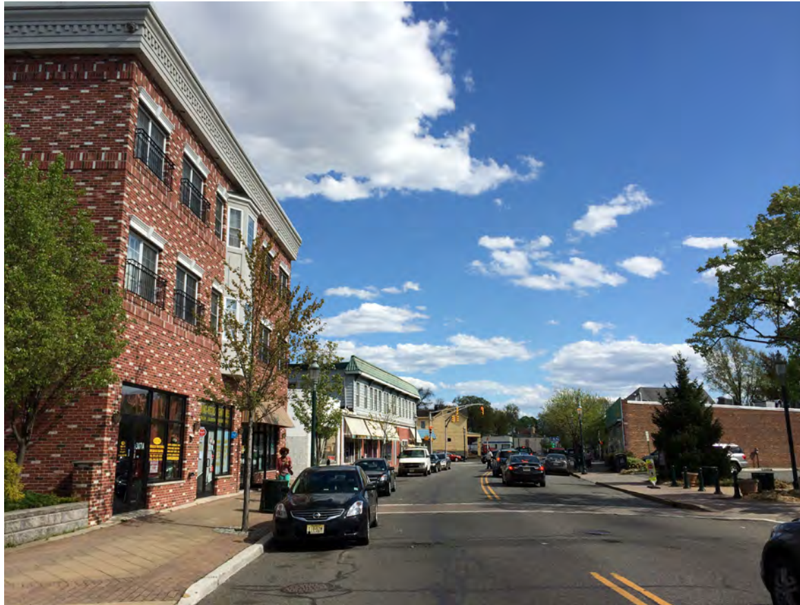
View of the Seton Village section of the Irvington Avenue Corridor
