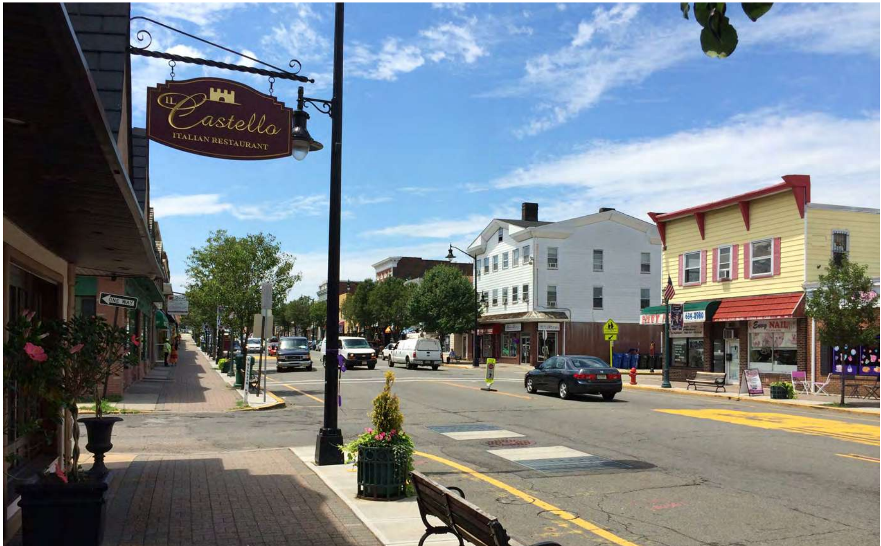
View of existing Main Street
