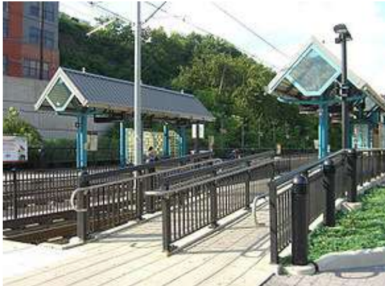
2nd Street HBLR Station
