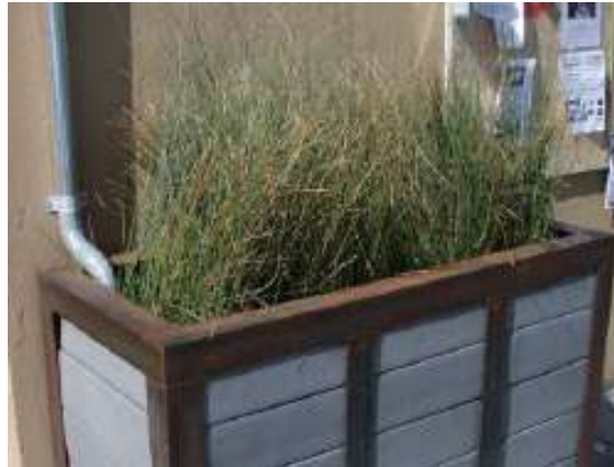
Stormwater Infiltration Planter
