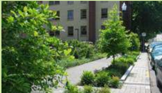
Stormwater Tree Pits
