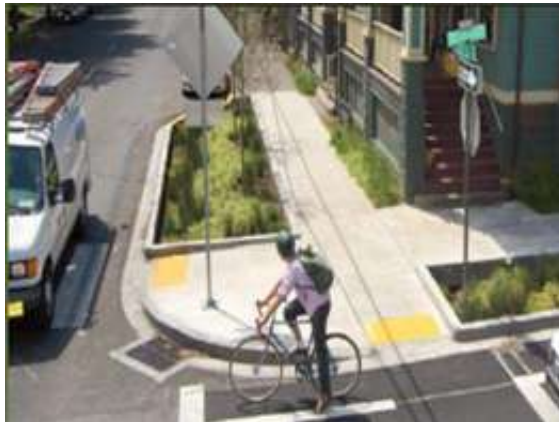
Rain Garden in right-of-way
