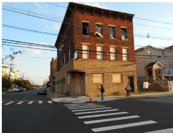
Image 27 Intersection of 2nd Street and Ripley Street
