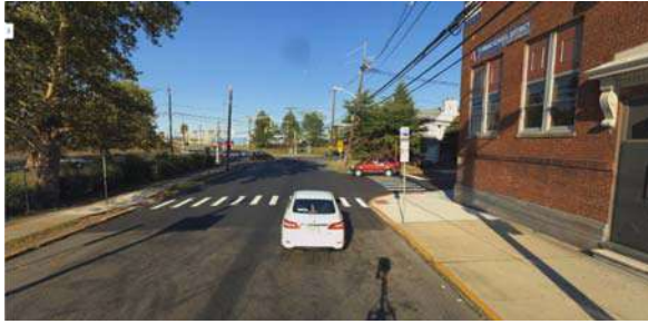
Image 15 School No. 13 Entrance
