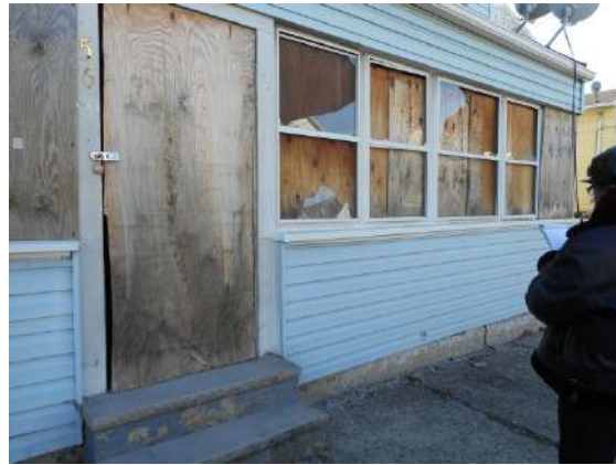
Image 59 Vacant Building on Geneva Street
