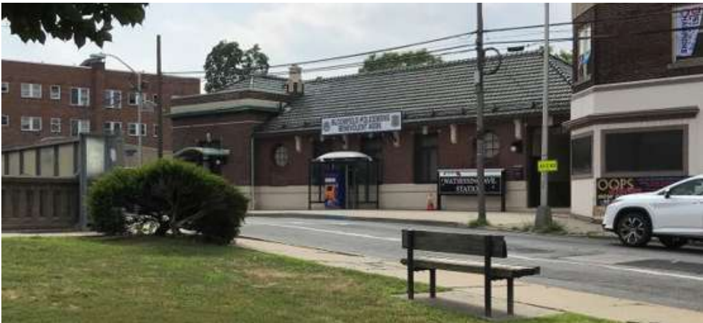
NJ TRANSIT Watsessing Avenue Rail Station (Bloomfield)
