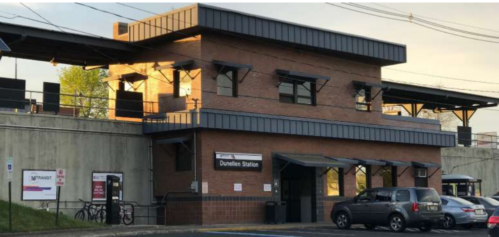
NJ TRANSIT Dunellen Rail Station
