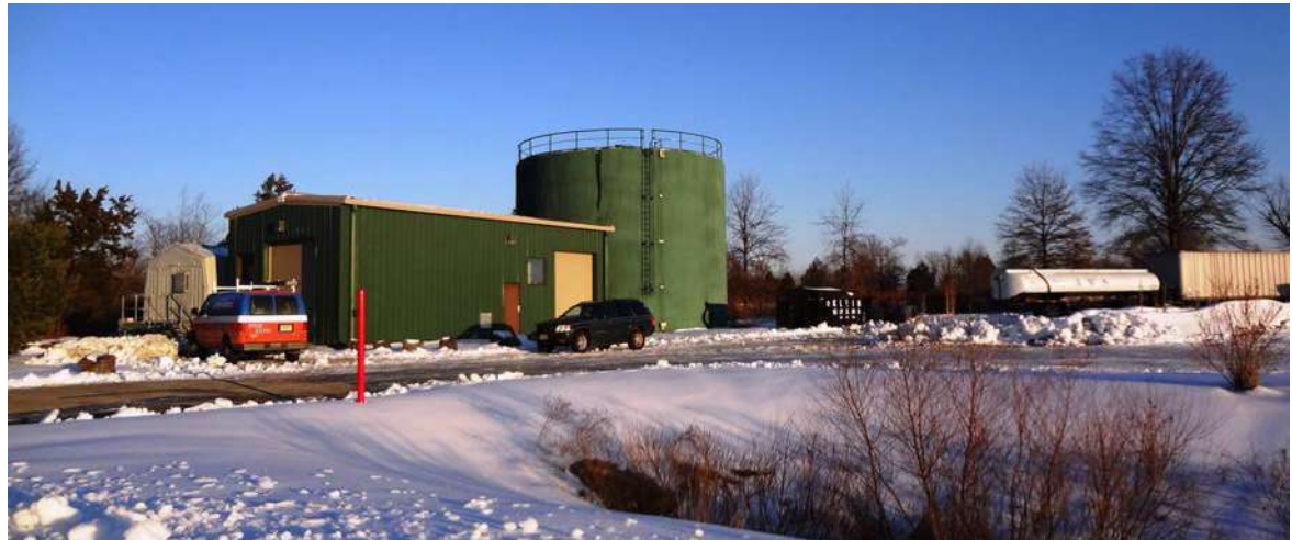
Treatment facility at business park
