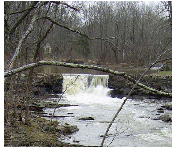
Milltown Road Falls in Kingwood
