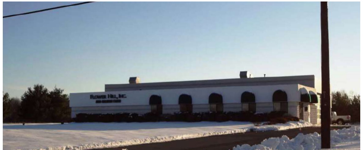
Commercial uses along Route 12
