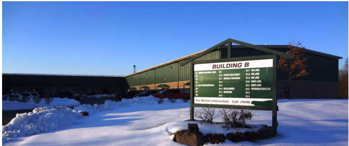
Route 12 Business Park
