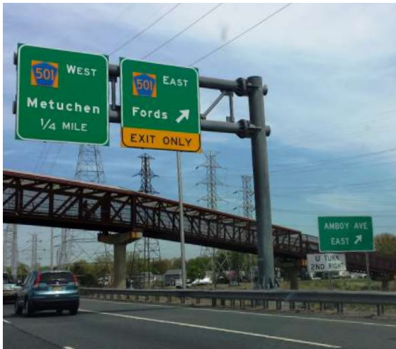
Greenway bridge over Route 1
