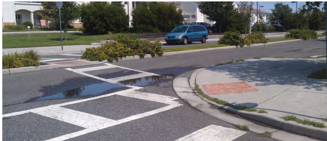
Add high visibility ladder crosswalks at all major intersections and other traffic calming on selective east-west streets will improve safe connections across the Study Area.
