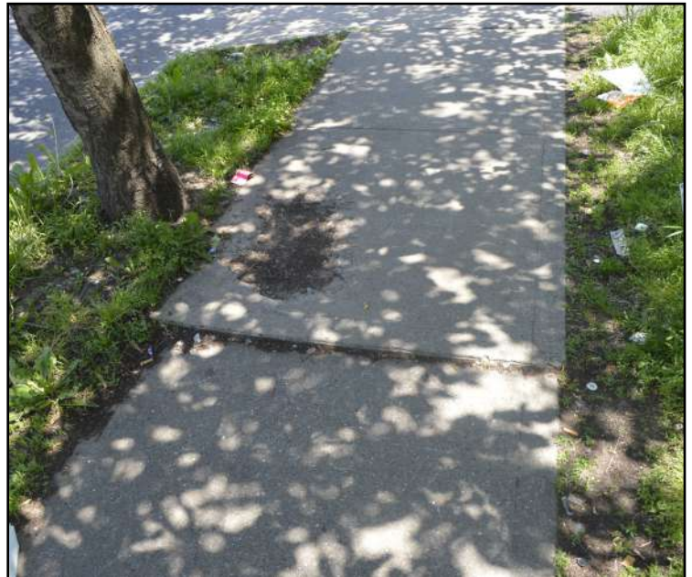
Uneven sidewalk on Orchard Street.
