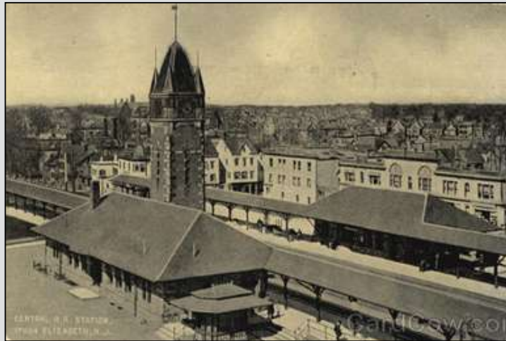
Figure 3: Early photo of the Elizabeth Midtown Station.
