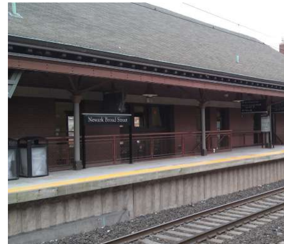
Newark Broad Street Station
