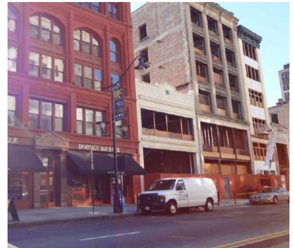
Construction in Downtown Newark
