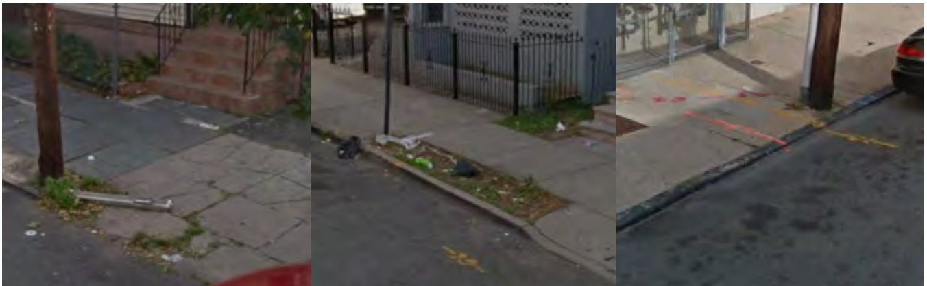
Figure 69. Existing sidewalks: Cracked driveway with bluestone slabs in background (L); 2-foot planting strip filled with litter (C); 3-inch granite curb height (R)
