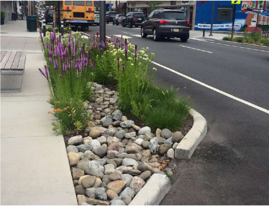
Stormwater Planter, Millburn, NJ
