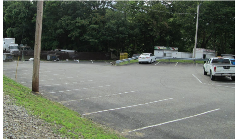
Parking lot viewed from freight line tracks
