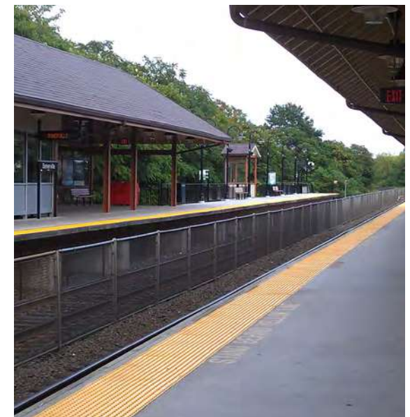
Somerville rail station
