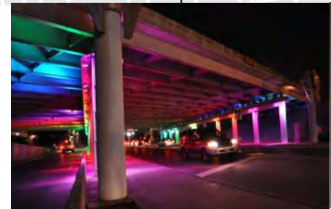
Route I-280 Underpass
