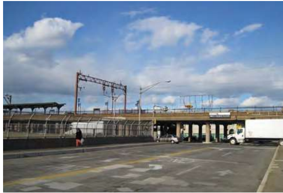
The overpass above I-280 in East Orange
