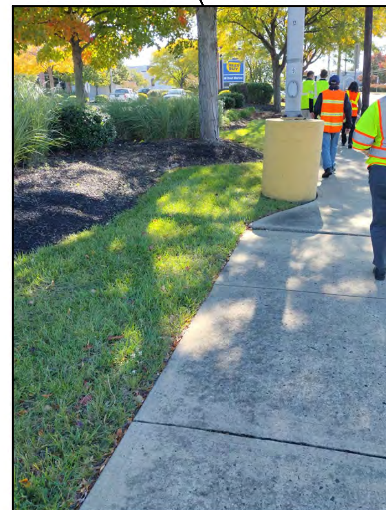
Sidewalk pathway cuts close to the roadway due to parking lot lighting
