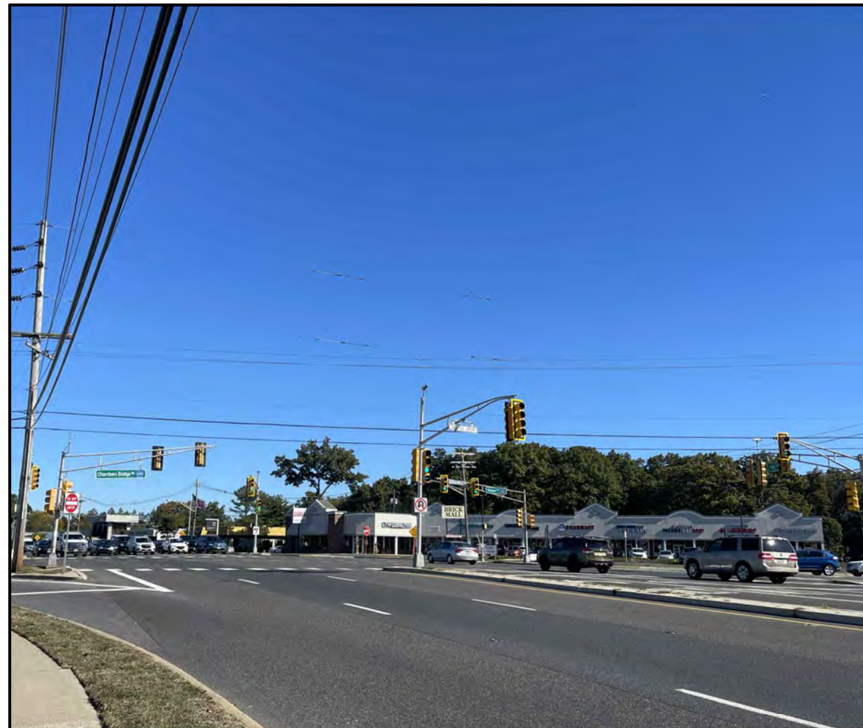
No lighting on traffic signal system
