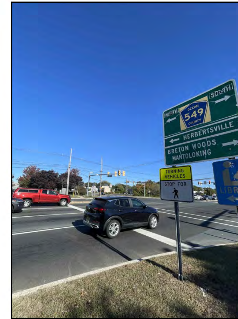
Worn and cracked signage
