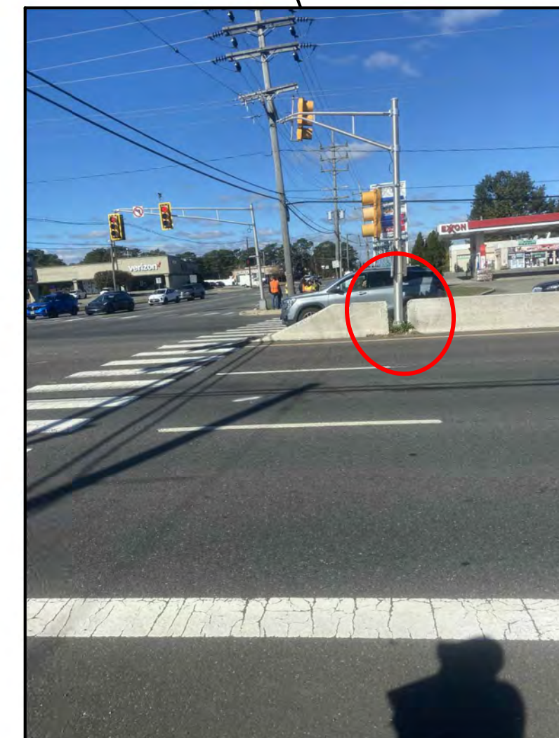
Signal pole between the concrete barrier
