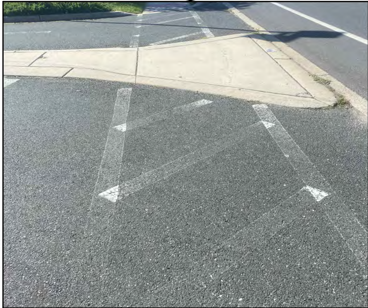
Faded Crosswalk striping
