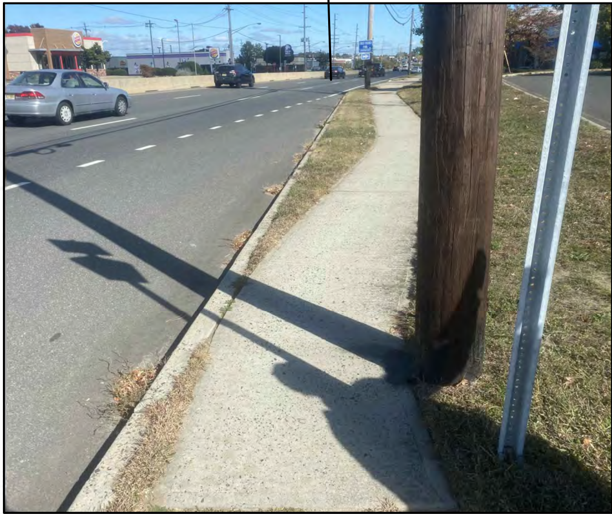
Utility pole restricts the sidewalk to be close to the roadway; Sidewalks is not 5' width
