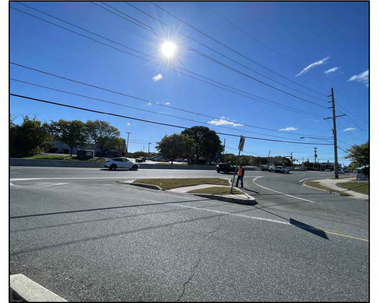
Faded striping; Missing crosswalk striping; No stop or yield signage at the turnlane
