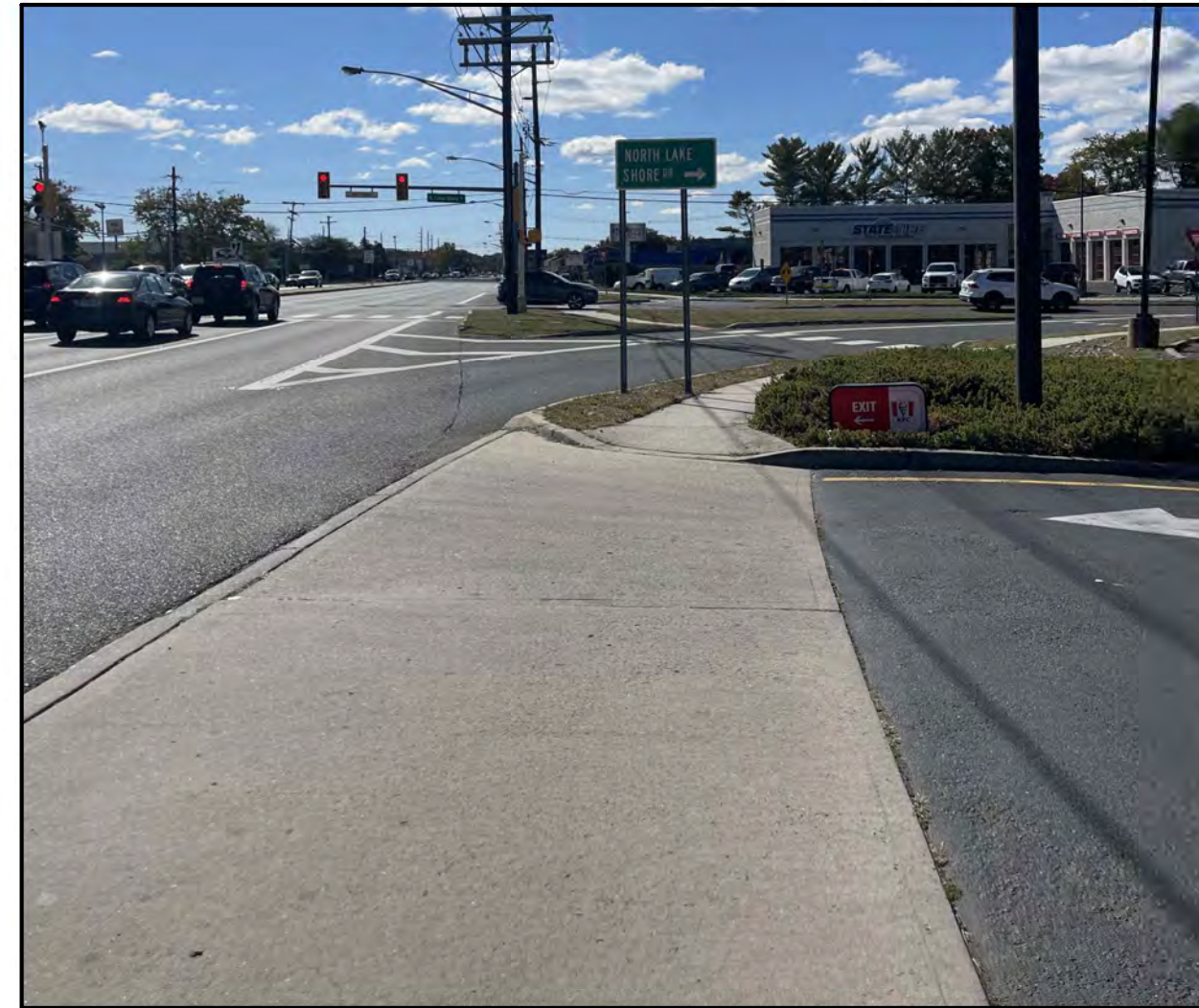
Driveway is directly off the ramp to Lakeshore Ave
