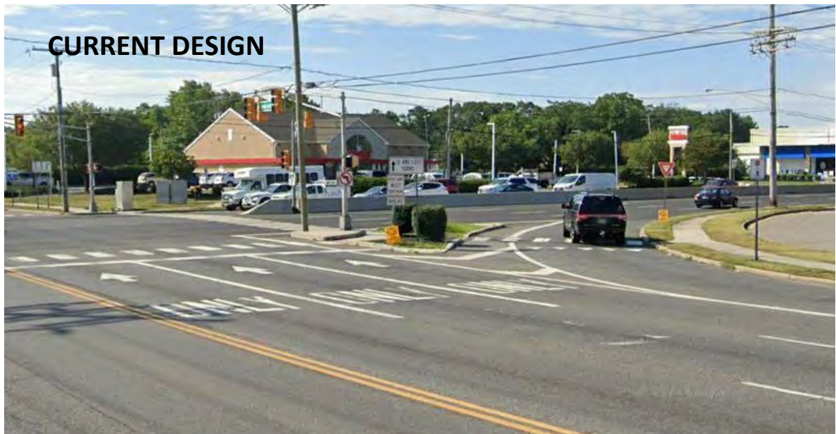
Figure 13 – Example of an Existing Channelized Right Turn Lane on the Brick Boulevard (Source: Google Street View)
