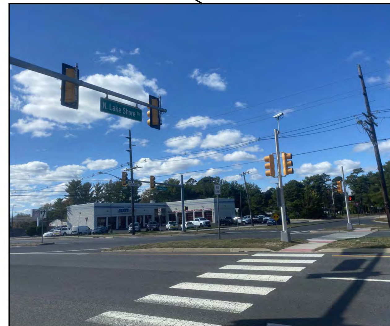
No lighting on the traffic signal equipment only on the utility poles on the SB side of Brick Boulevard
