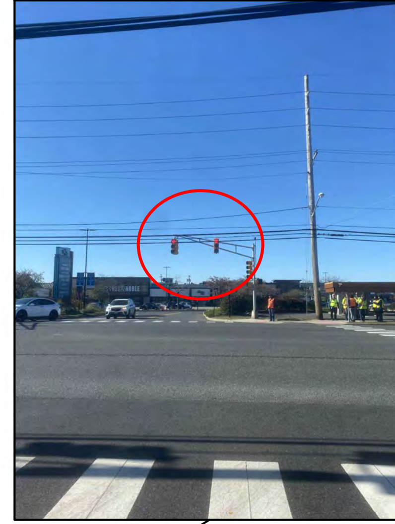
Utility wires obstructing traffic signal view
