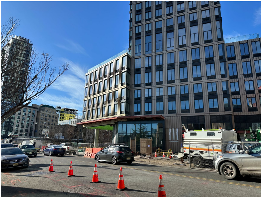
Figure 25: New residential developments under construction in Journal Square neighborhood
