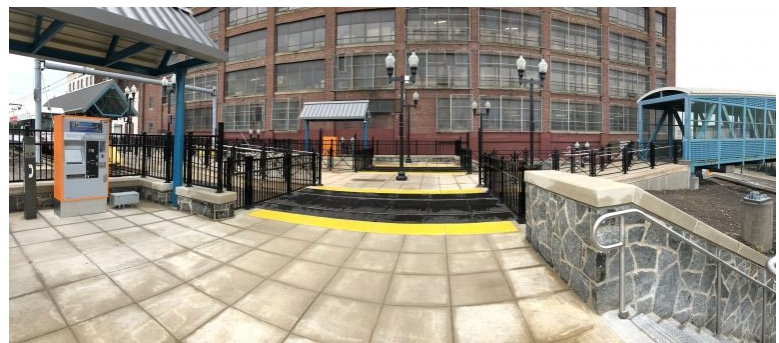
Figure 41: West Side Ave Light Rail Platforms
