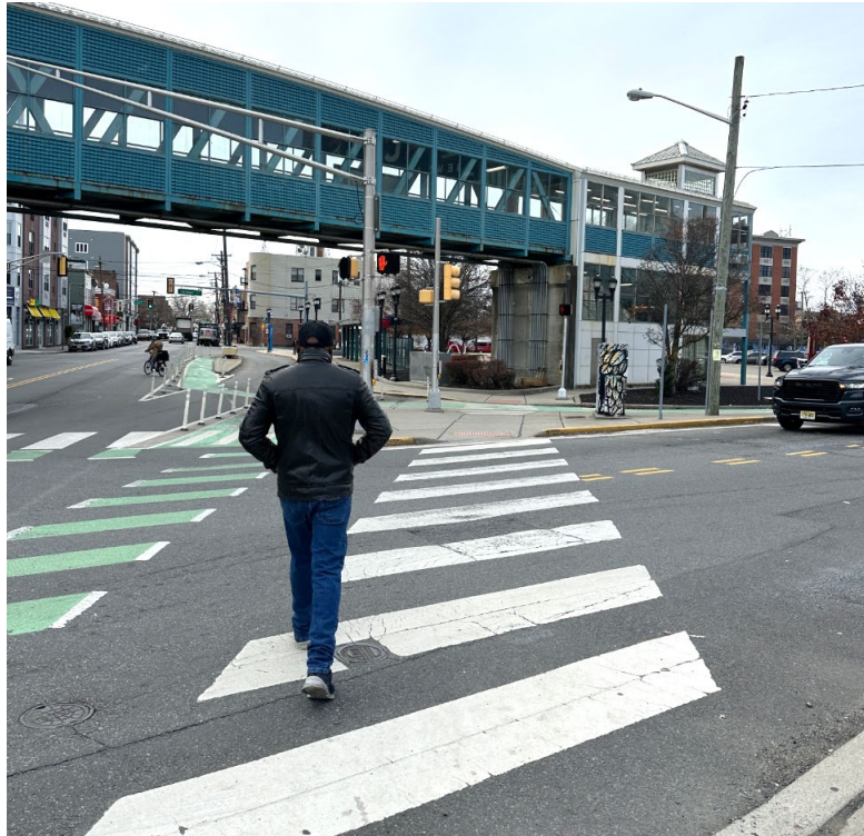
Figure 15: West Side Avenue, nearby Hudson Bergen Light Rail Station
