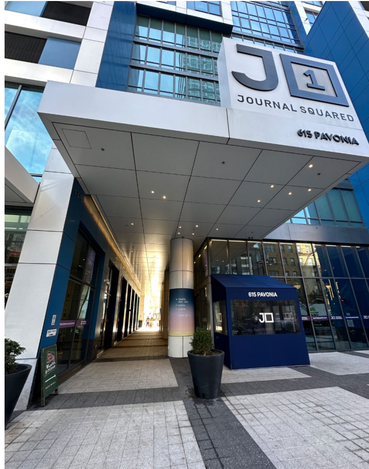
Figure 21: Access to Journal Square Transportation Center through Journal Squared Development
