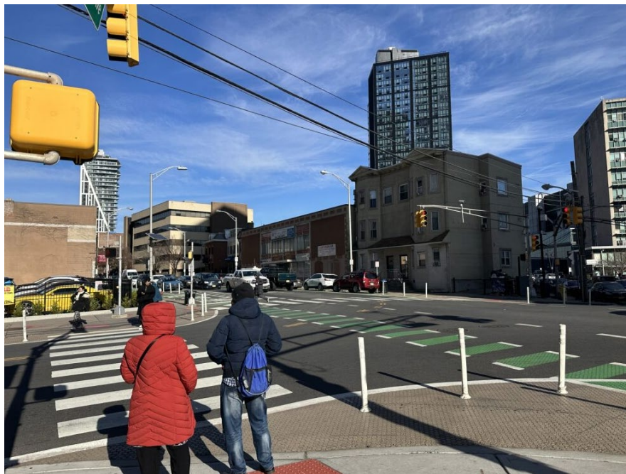
Figure 52: Summit Avenue / Central Avenue / Pavonia Avenue intersection today
