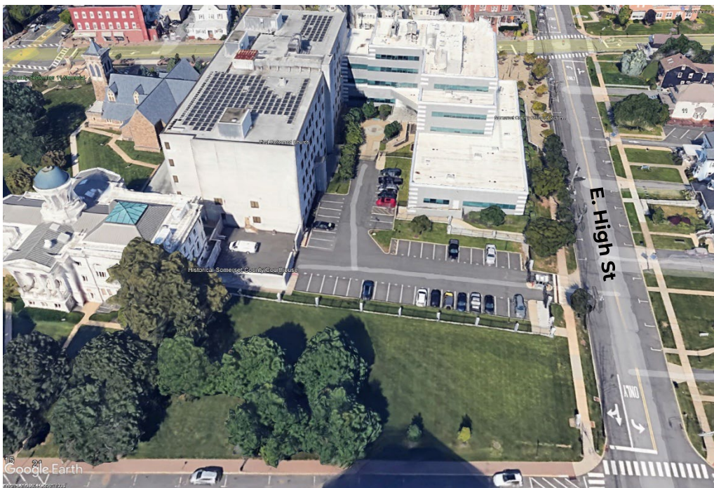
Figure 16: Court House Aerial View
