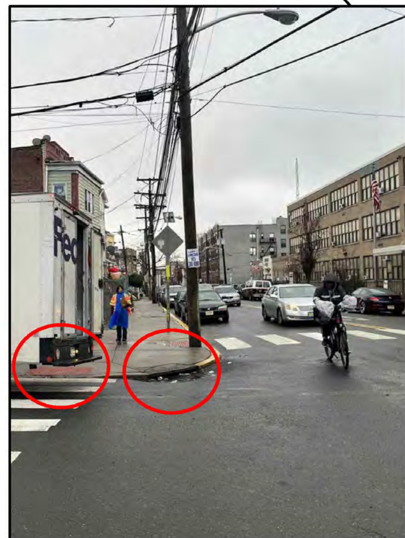
Truck parked blocking the crosswalk; damaged sidewalk around the inlet
