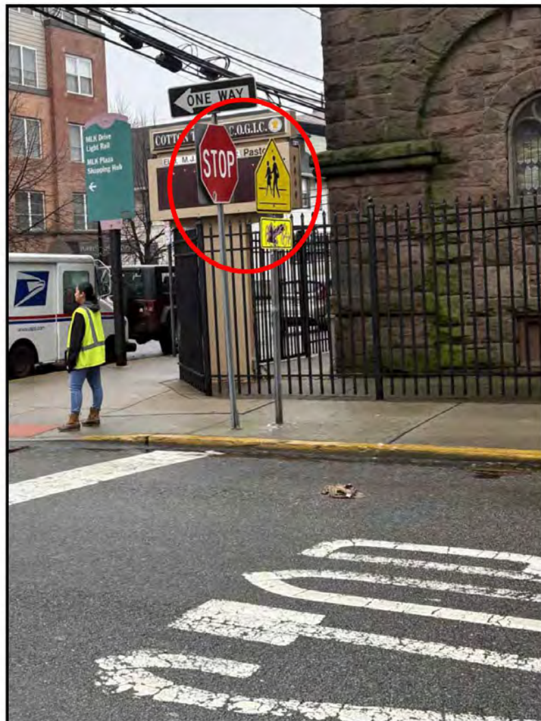
Worn traffic markings; outdated school crossing sign; signs are not MUTCD compliant
