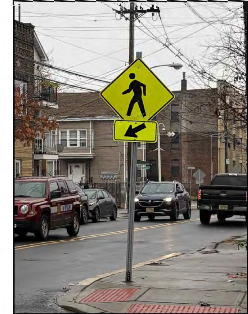
Crosswalk sign is not at the proper height
