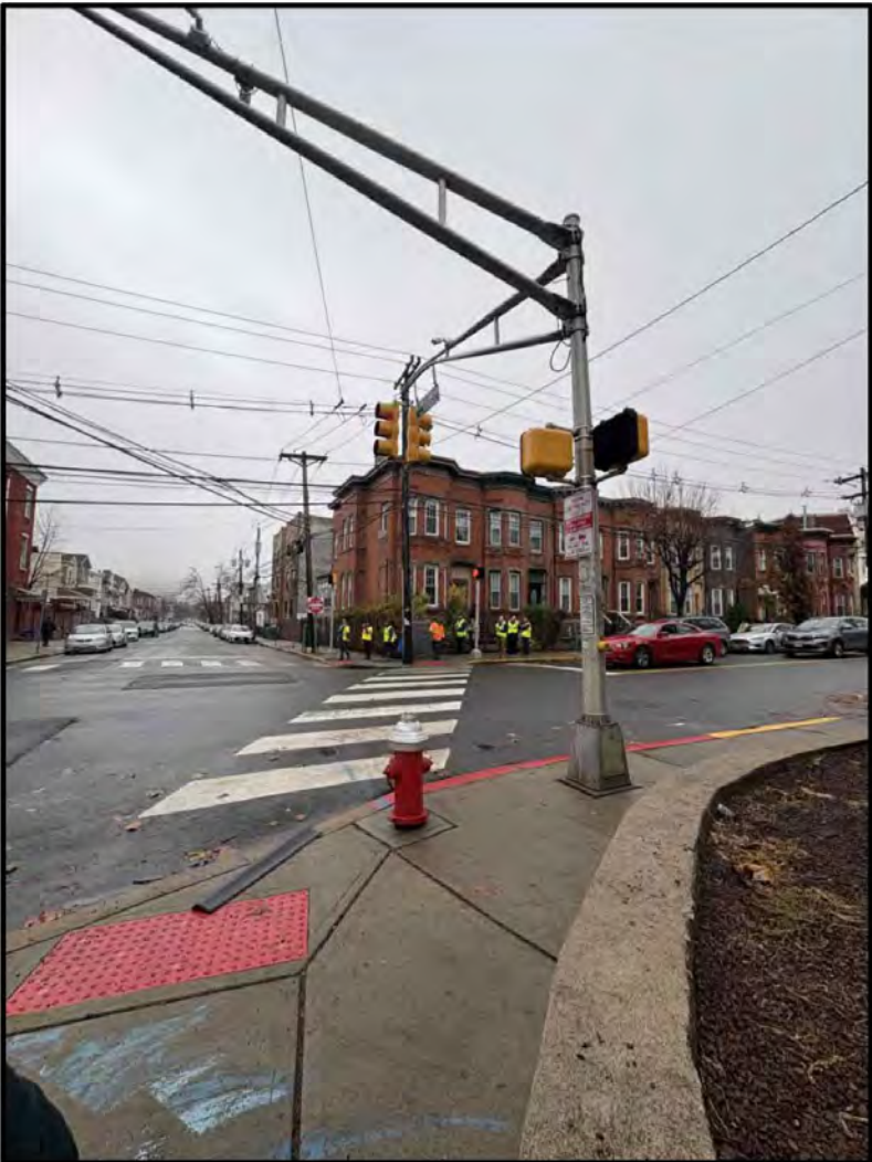
Crosswalk is skewed
