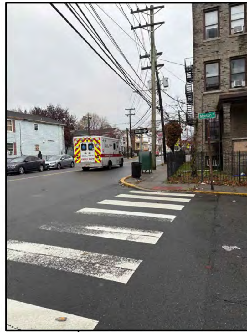
Faded crosswalk striping
