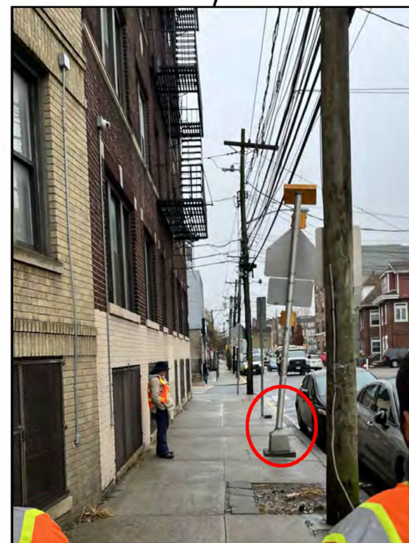
Flashing school crossing sign is tilted
