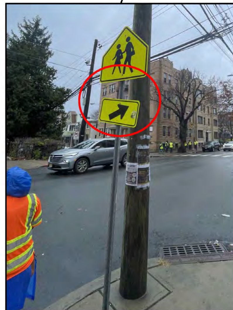
Crosswalk sign broken and facing the wrong direction
