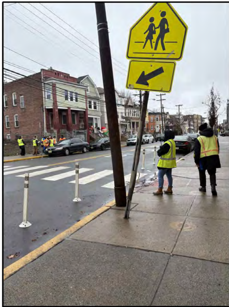
Sign and sign post on an angle
