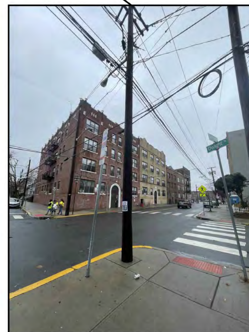
Street sign pole is bent
