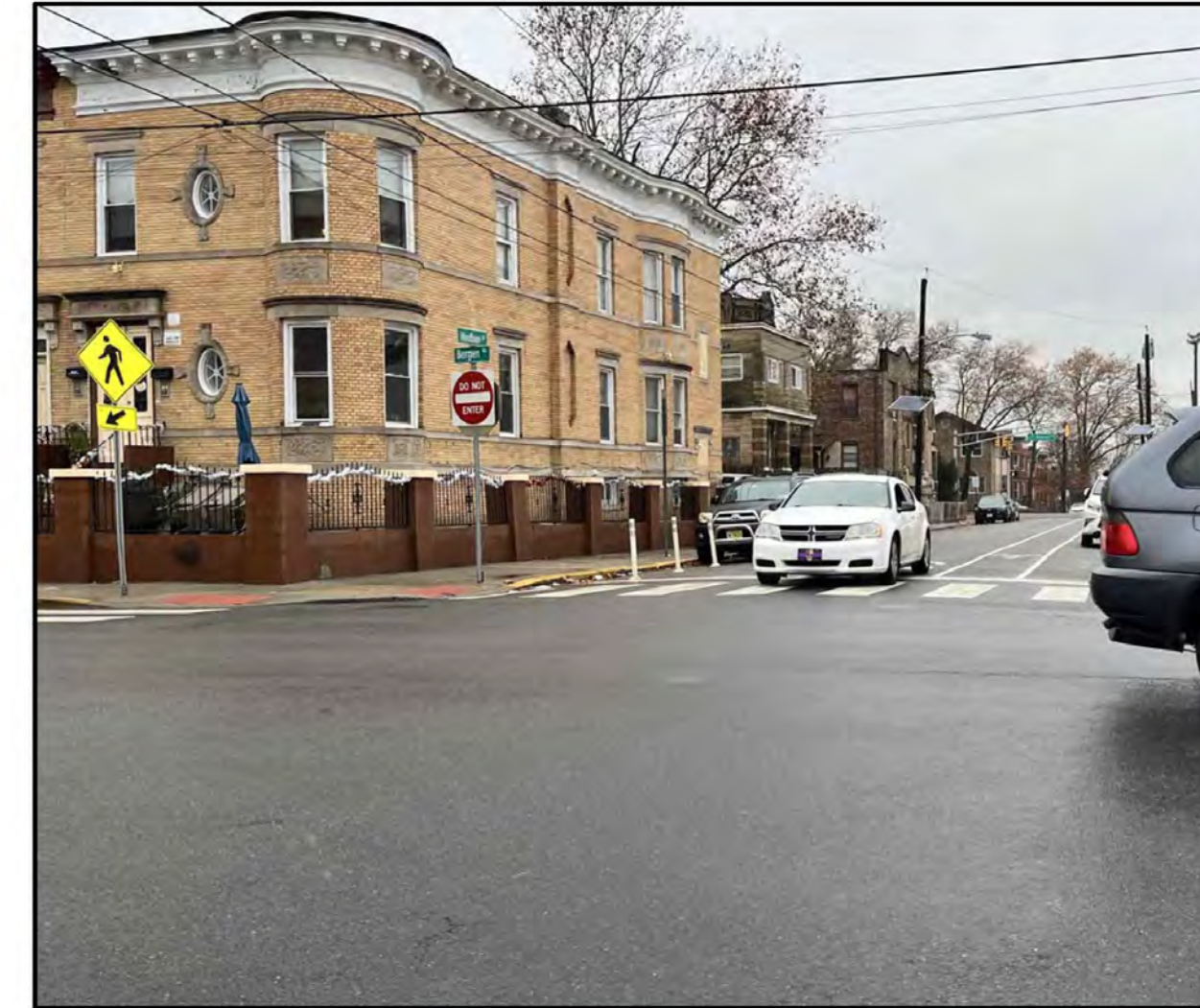
Fence obstructing the sight distance
