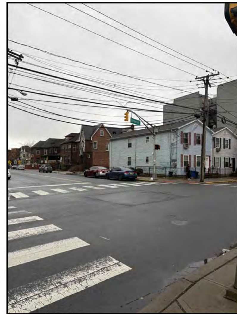
Worn crosswalk striping
