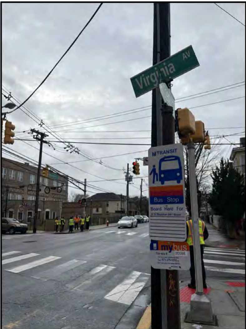
Broken sign; low signage
