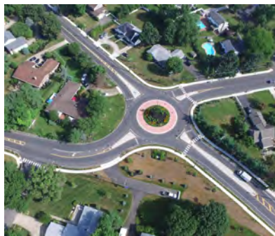
Roundabout, Cinnaminson Township, Burlington County
