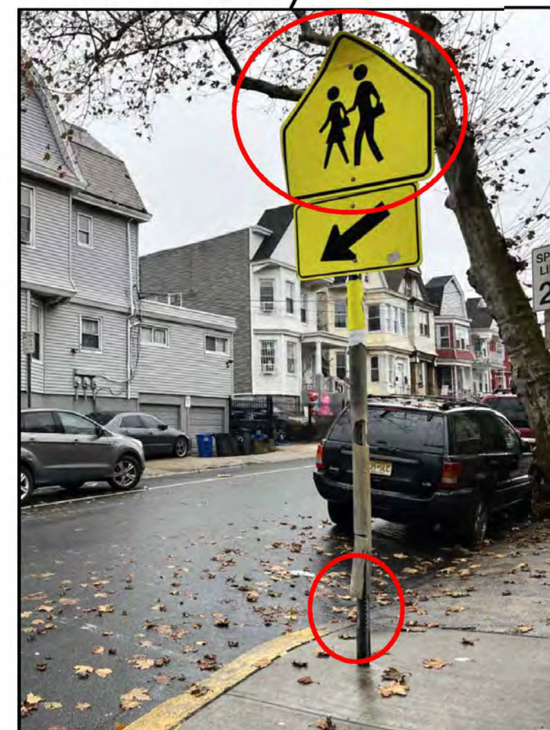
Bent sign; Sign post is broken
