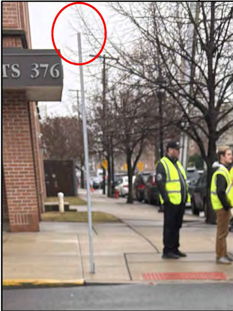
Missing sign; no crosswalk striping
