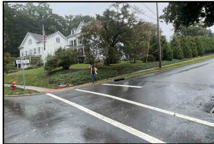
No edgeline and centerline markings; Narrow sidewalk; Sightline issues due to the intersection geometry and landscaping elements
