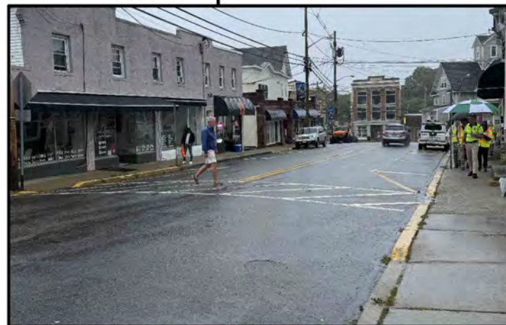
Faded crosswalk; Missing ADA curb ramps
