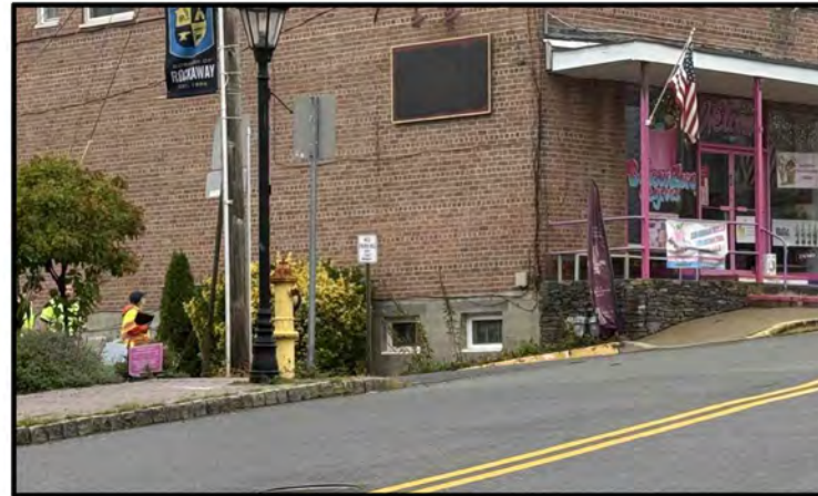
Sidewalk obstructed due to utility poles and fire hydrants; No crosswalk; Missing ADA compliant curb ramps
