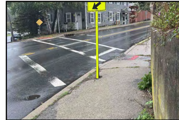
Faded crosswalk; Debris accumulated at curb ramp; Incorrect stop bar location
