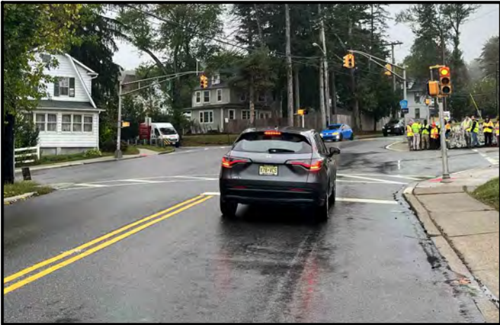
No tracks marks; No buffer between sidewalk and vehicle lane; Narrow sidewalk
