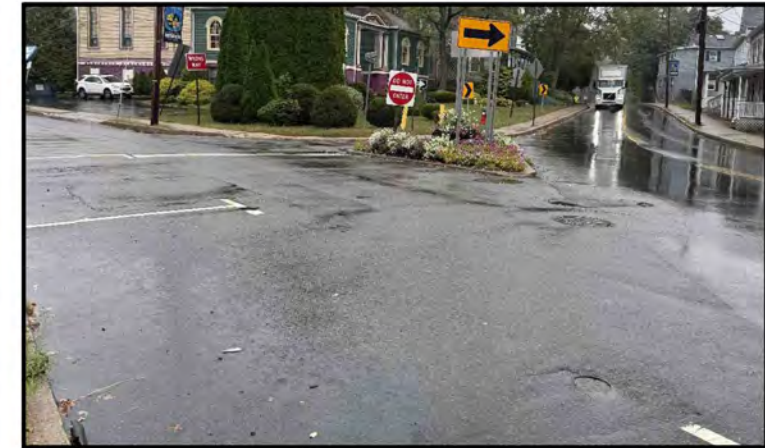
Street parking at the intersection; Illegible street name signs; Sightline obstruction due to the landscaping island
