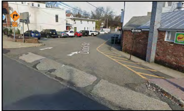
No crosswalk; No ADA compliant curb ramps
