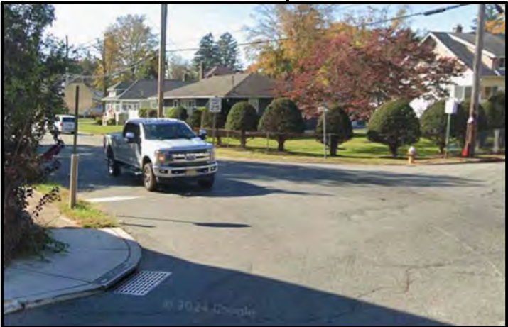
No crosswalk; No ADA compliant curb ramps; No edgeline and centerline markings
