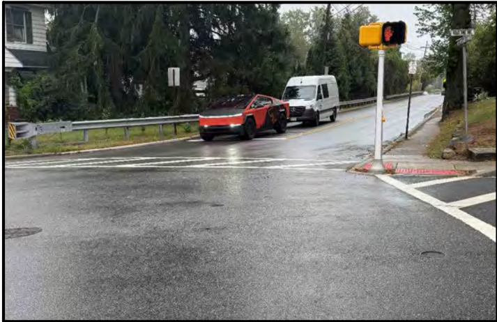
Illegible street name signs; No sidewalk on EB Hoagland Avenue
