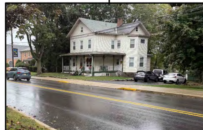
No driveway warning sign
