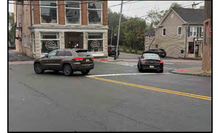
Sightline issues due to the existing corner building
