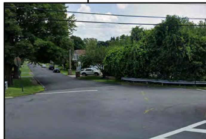
No crosswalk; No centerline and edgeline markings; Sightline issues due to intersection geometry; No track marks
