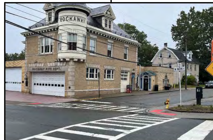
Fire hydrant obstructing the sidewalk; Illegible street name signs
