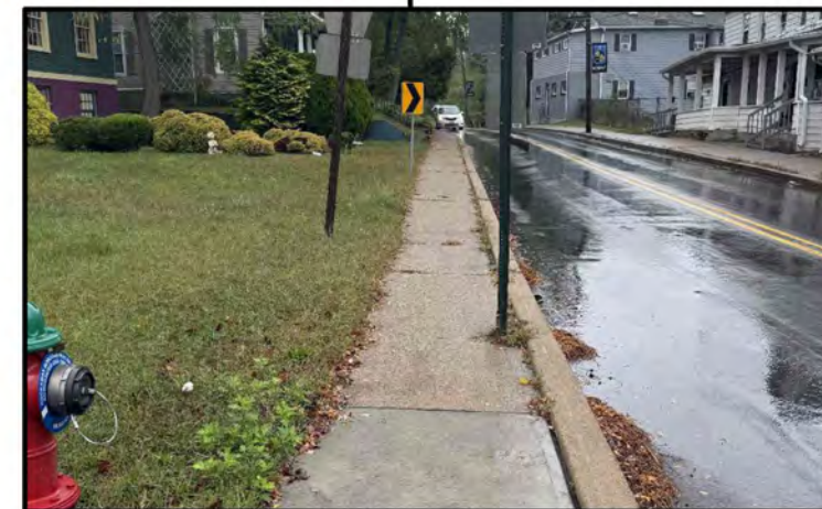
Narrow sidewalk; Roadway sign obstructing the sidewalk
