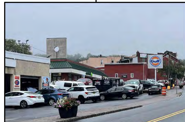
Poor driveway access mangement of the commercial establishments; Missing no left turn signs
