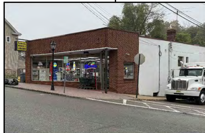
Missing ADA compliant curb ramp; Faded crosswalk
