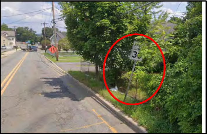
Speed sign bent and hidden due to the overgrown vegetation; No sidewalk
