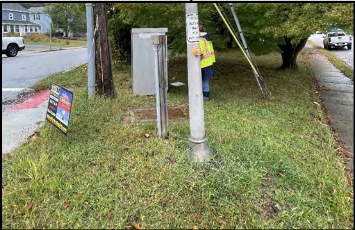
Non ADA compliant pedestrian signal push button location
