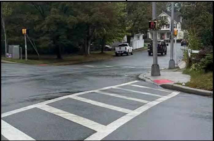
No sidewalk; No edgeline and centerline markings
