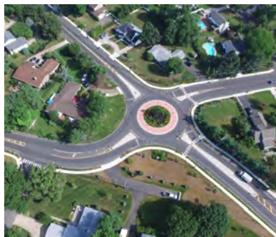
Roundabout, Cinnaminson Township, Burlington County
