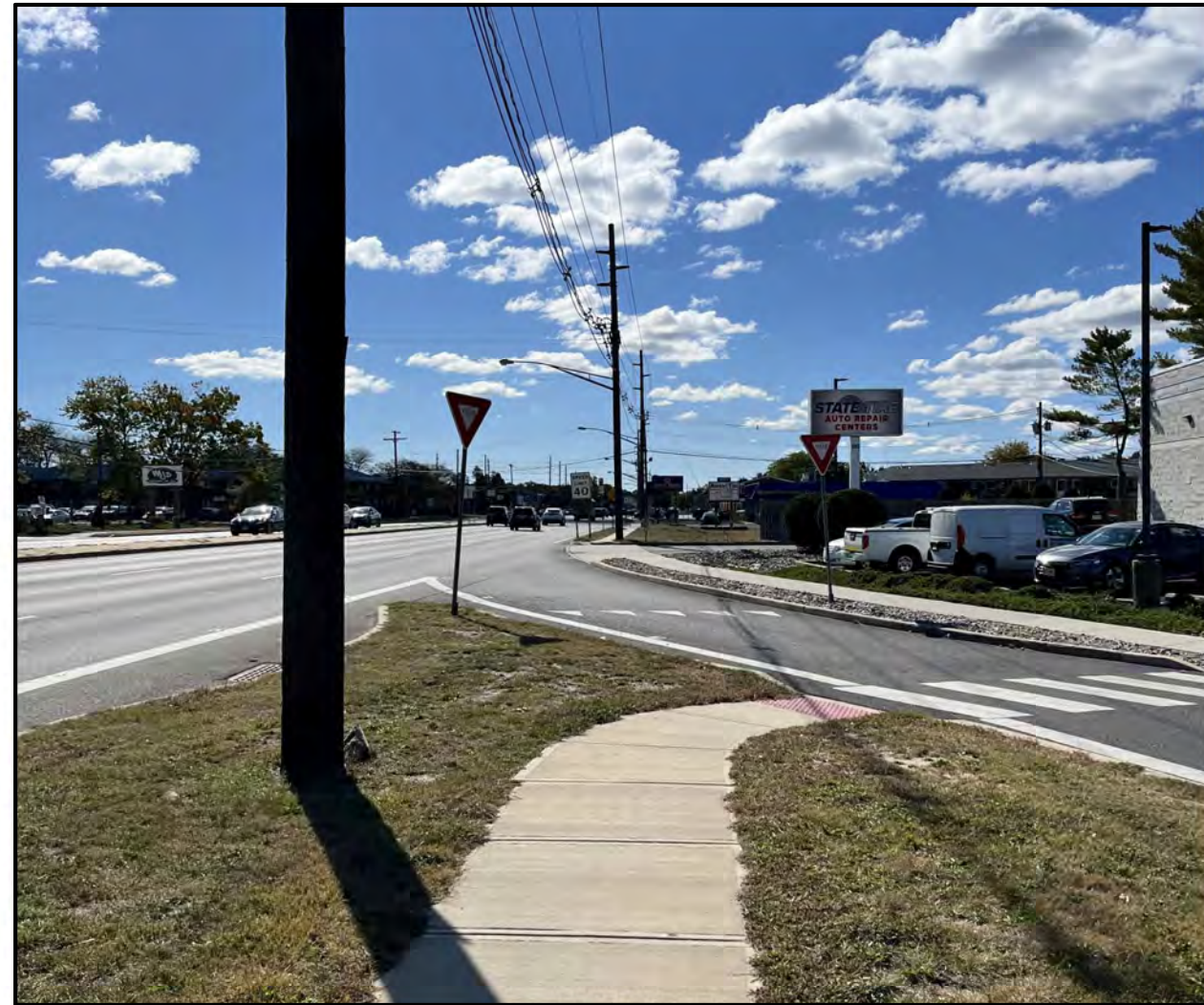
Congestion on Brick Boulevard SB is due to the decrease from 3 lanes to 2 lanes
