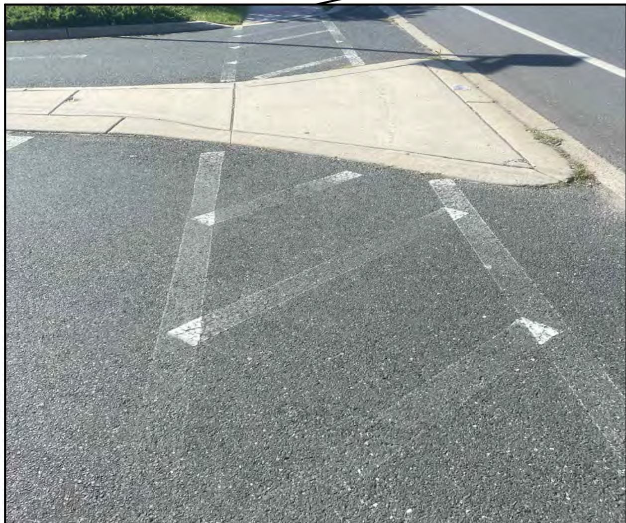
Faded Crosswalk striping
