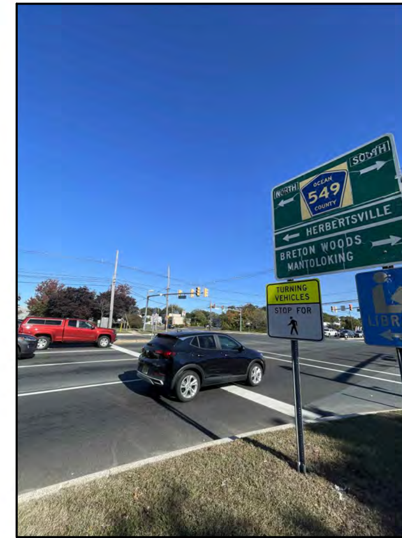
Worn and cracked signage
