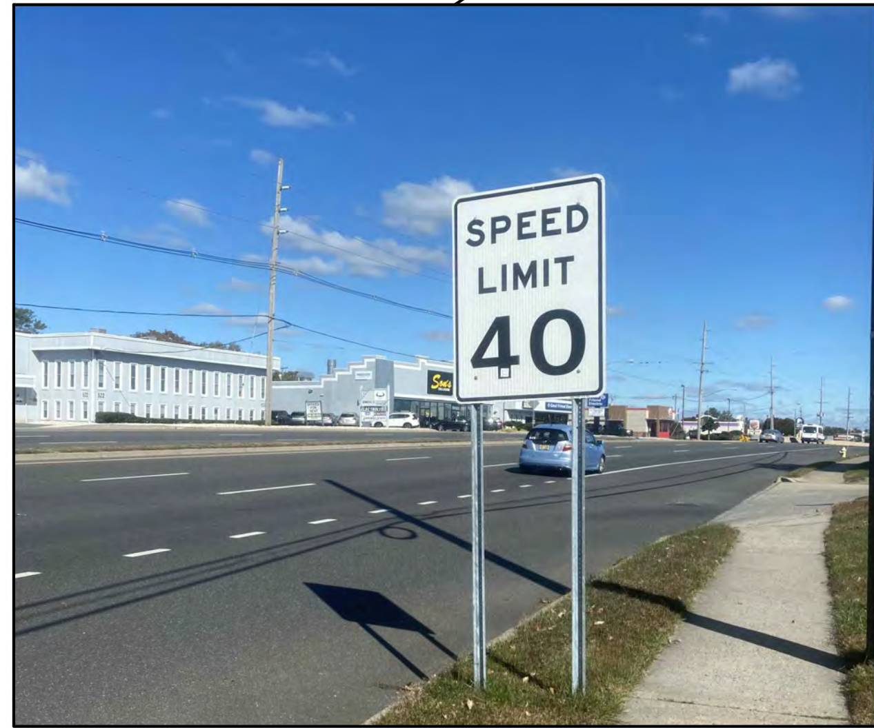
Low visibility of the speed limit sign due to placement
