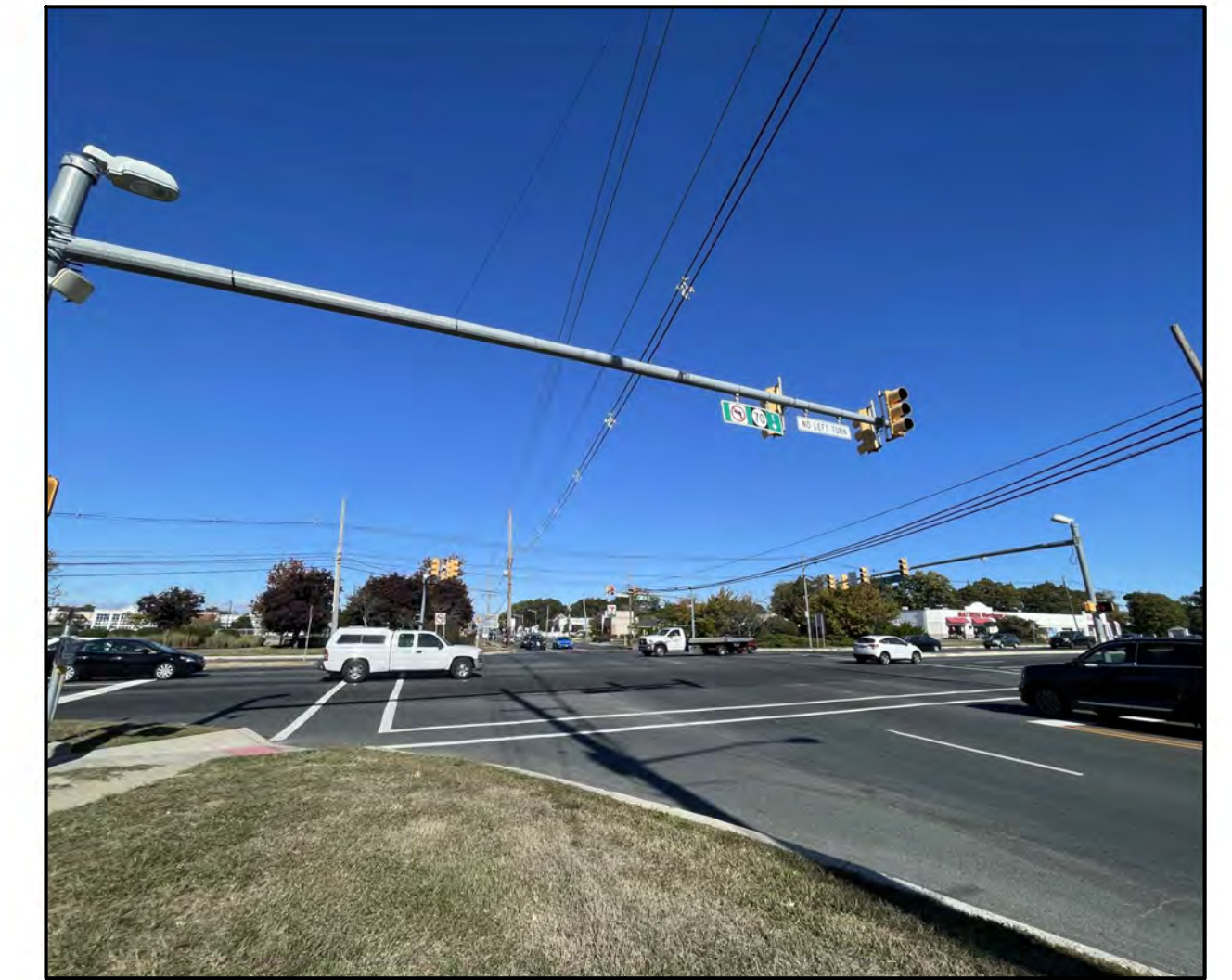
No lighting at the intersection; No backplates
