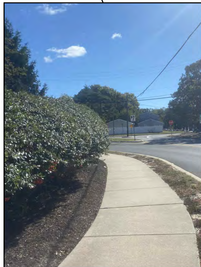
Vegetation obstructing the sight of pedestrians using the crosswalk
