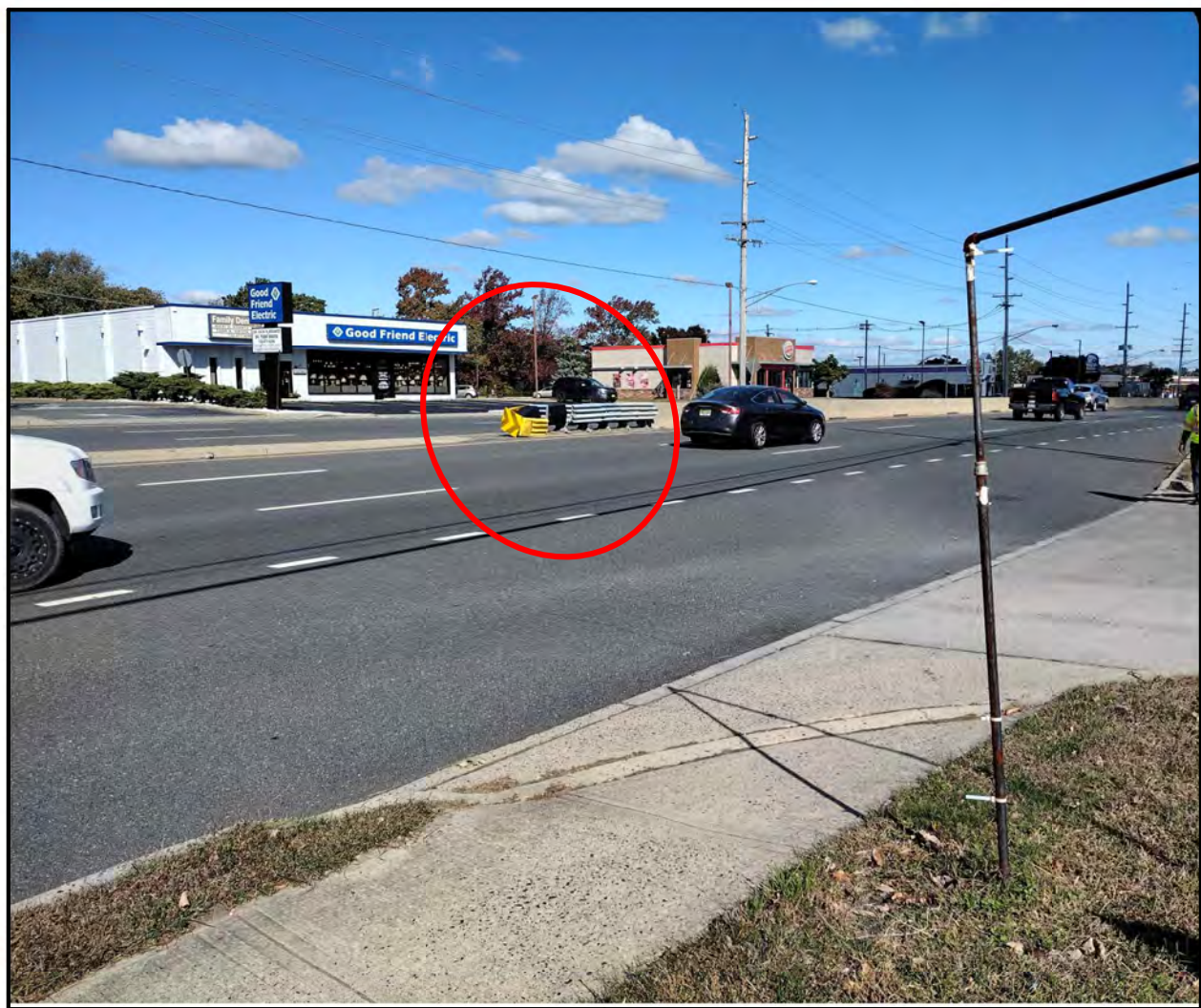
Broken barrier at the start of the concrete dividers
