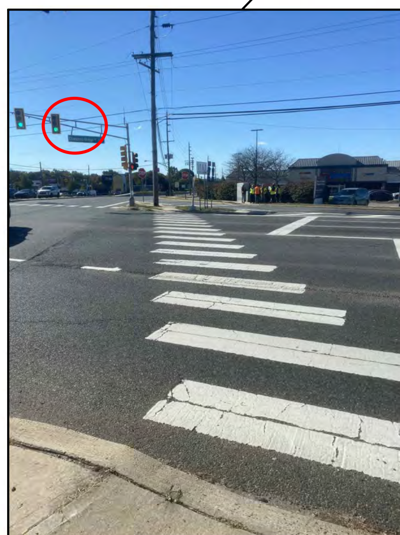
Broken traffic signal equipment
