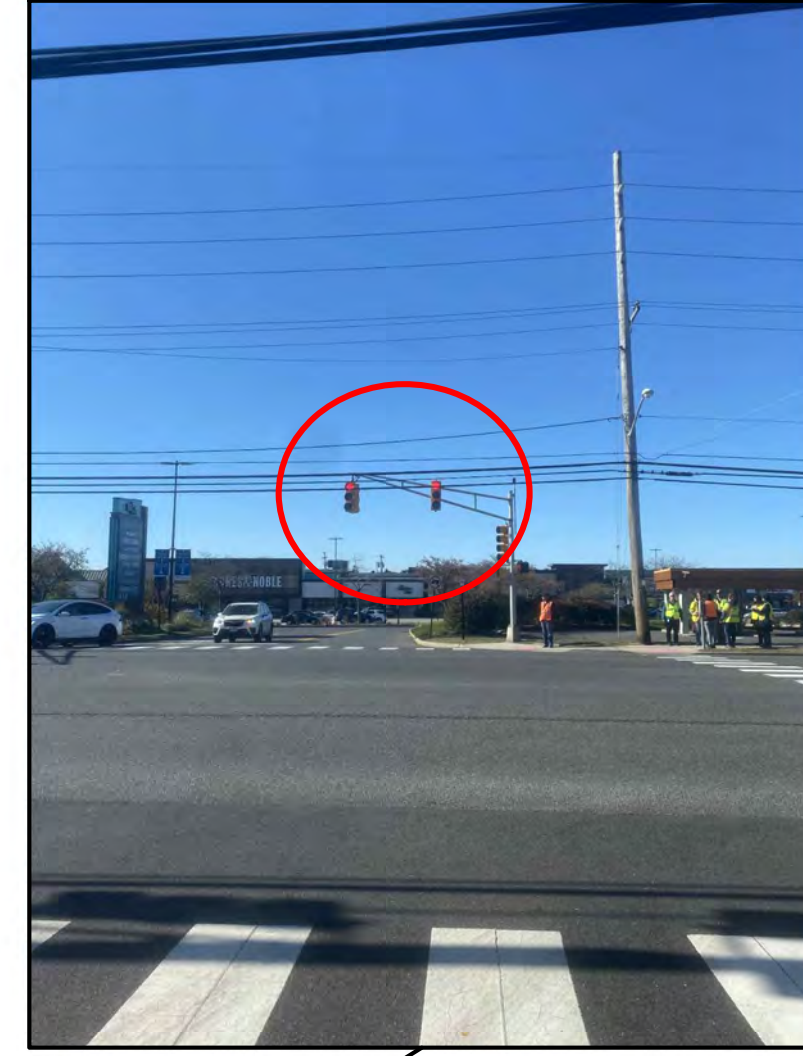
Utility wires obstructing traffic signal view
