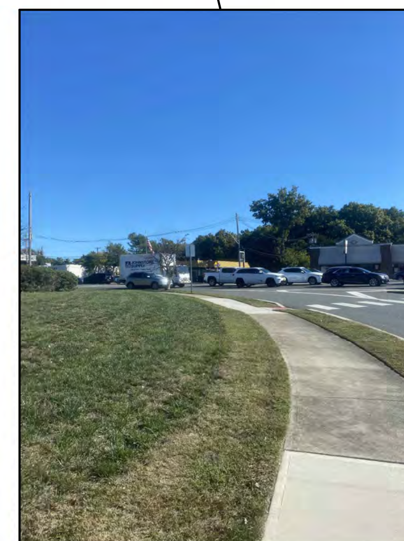
Turning radii obstructs pedestrian views of the farther crosswalk
