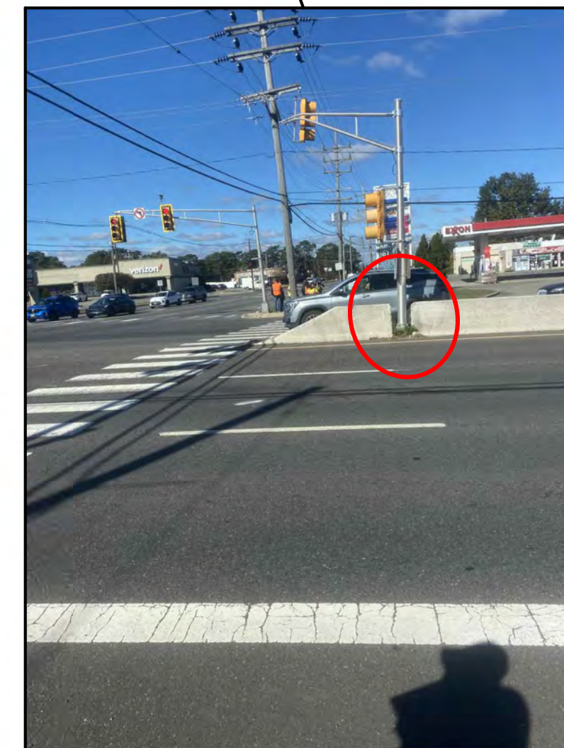
Signal pole between the concrete barrier
