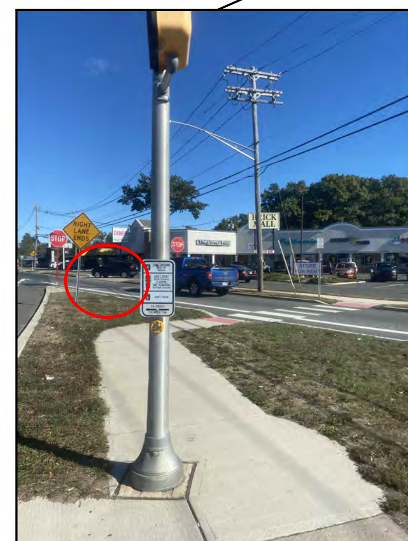
Driveway close to the the ramp
