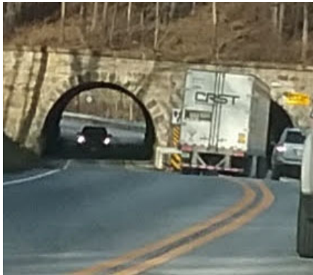
Truck Stuck in CR 519 Tunnel
