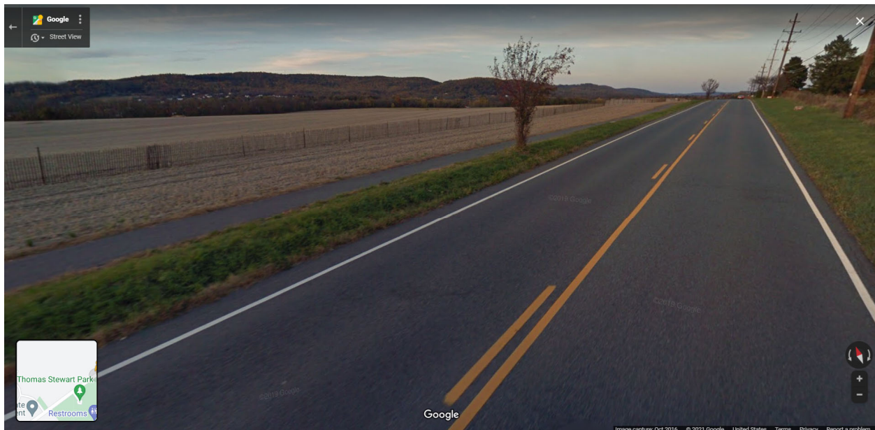
CR 638 Sidepath, Greenwich Township
